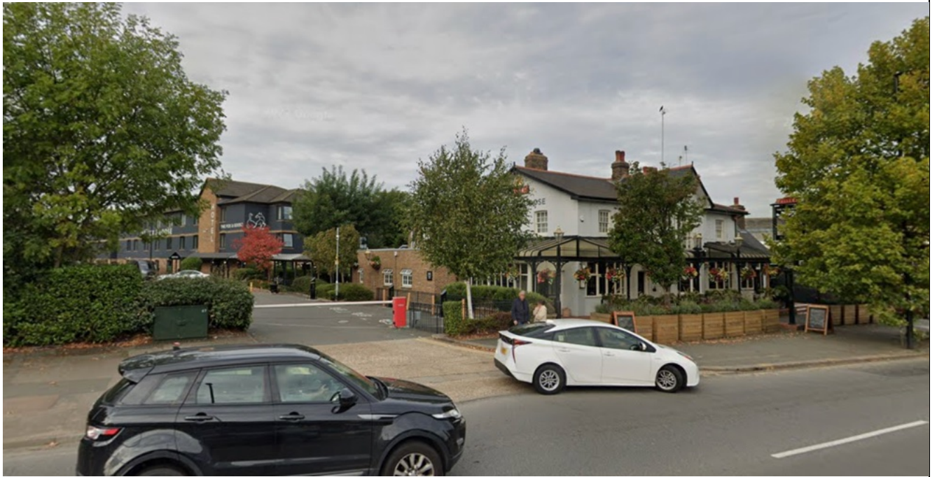
Image 5: View of the application site taken from the 'Fox and Goose' hotel. The 'Big Yellow Storage' unit is to the rear and clearly not visible from Hangar Lane (Source: Google Maps)
