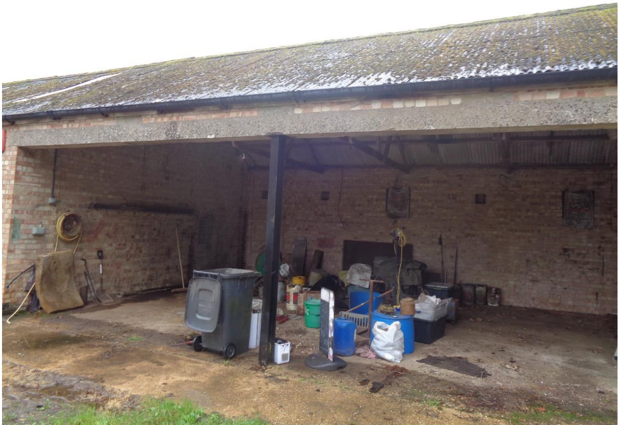
Northern elevation where the bays are to be enclosed
