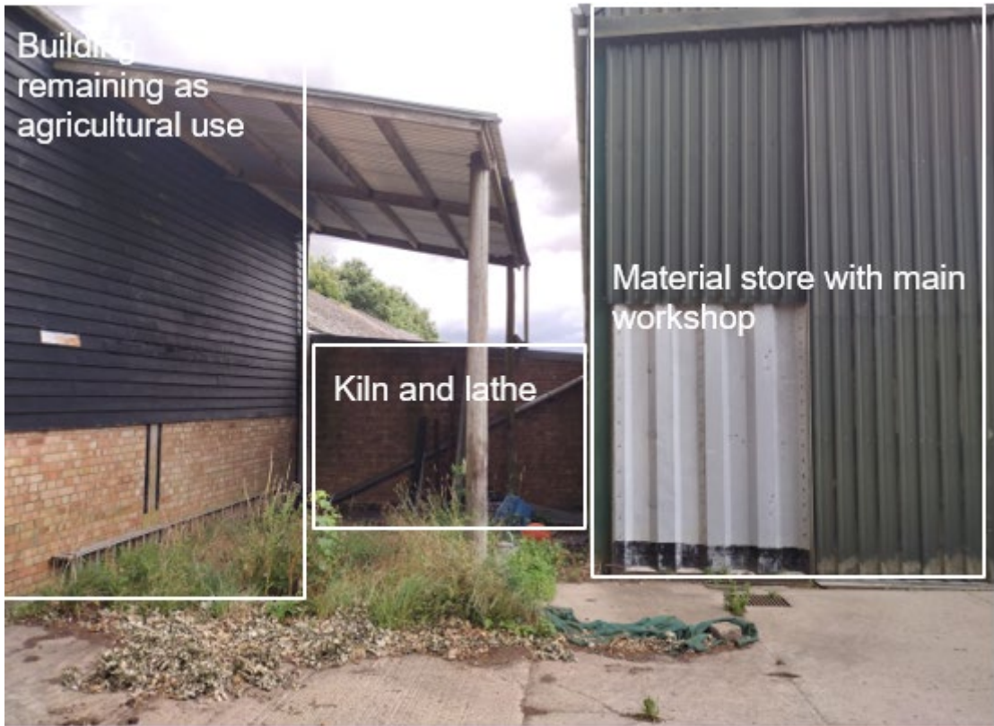
Figure 6 – View of existing buildings and proposed uses
