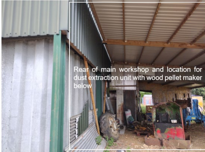
Figure 7 – View of existing buildings and proposed uses
