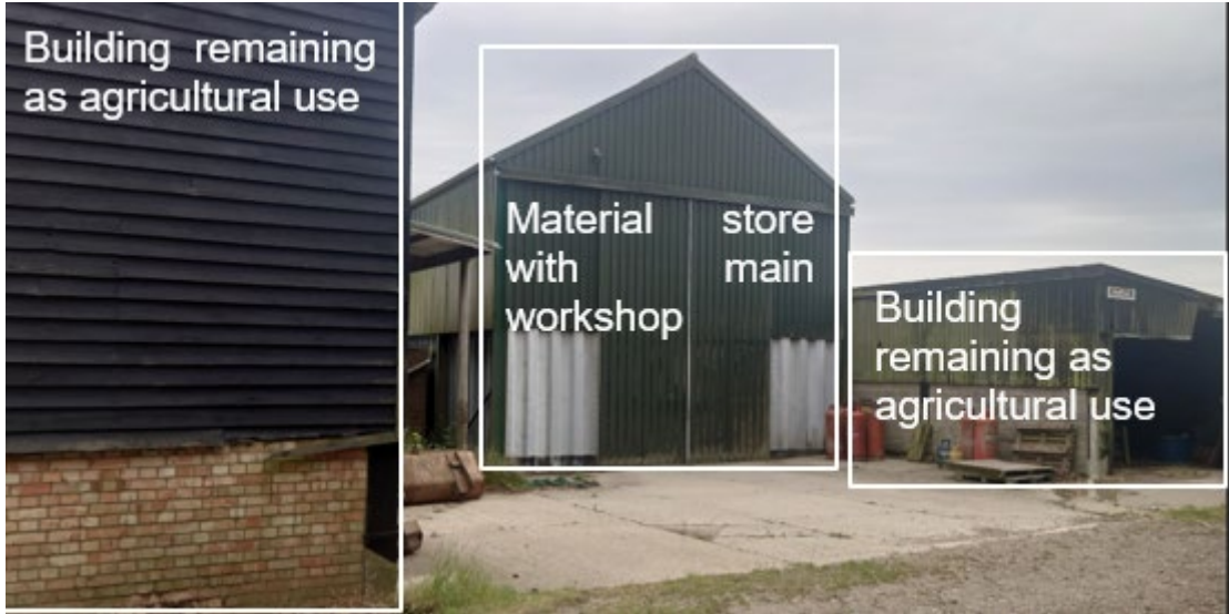
Figure 5 – View of existing buildings and proposed uses
