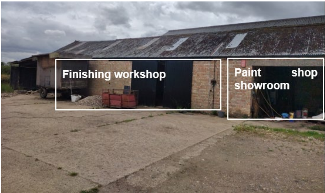
Figure 4 – View of existing buildings and proposed uses
