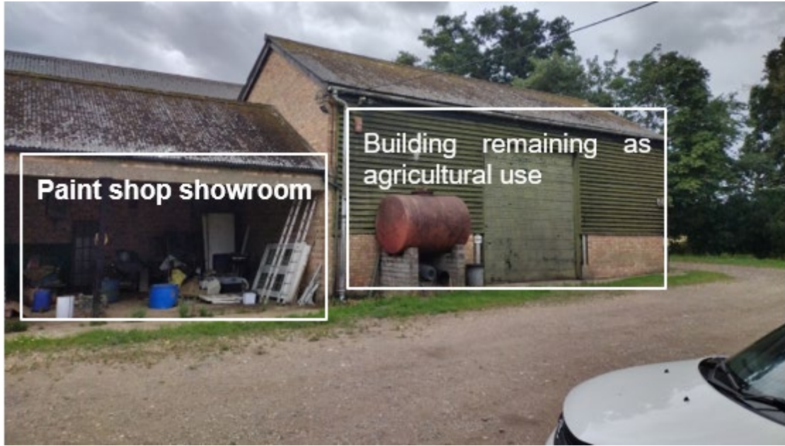
Figure 3 – View of existing buildings and proposed uses
