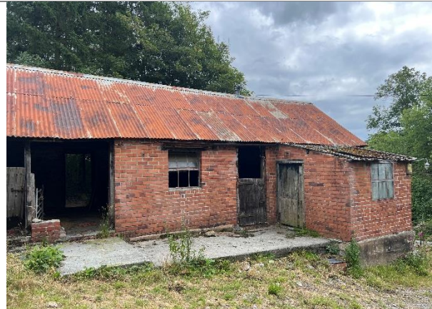
Western elevation of the main building.
