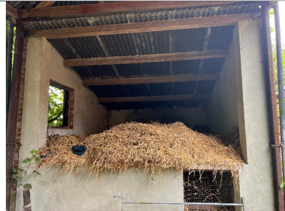
Lean-to shelter adjoined to the east of the main building.
