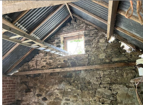
Window present on the northern gable of the main building.
