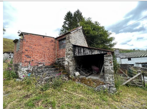
Southern elevation with view of lean-to garage section.
