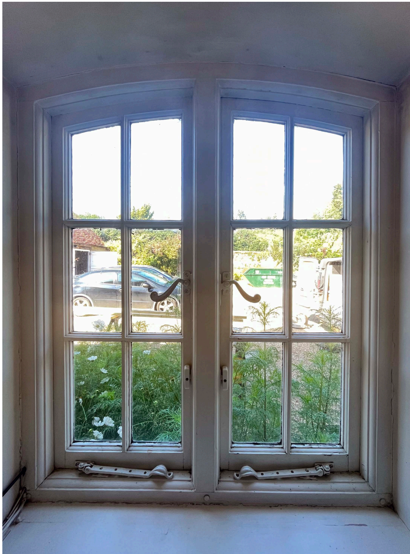
Image: Internal view of example casement window (G5).
