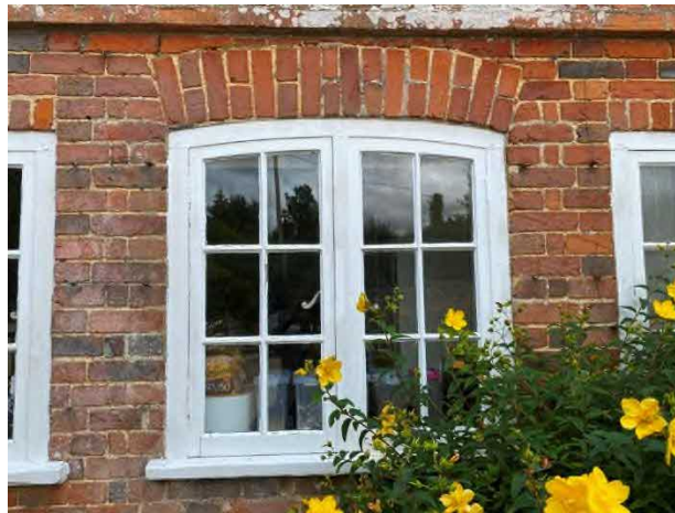
Figure 22: Exterior of window G2
