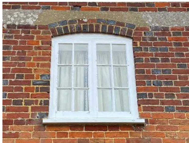
Figure 36: Exterior of window F5
