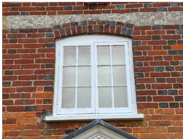
Figure 33: Exterior of window F3
