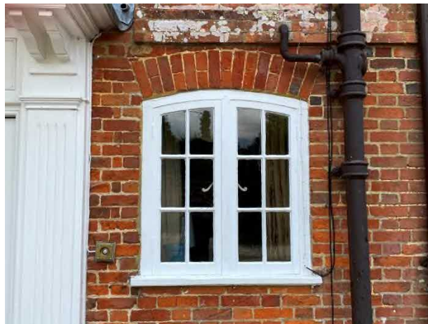
Figure 24: Exterior of window G5
