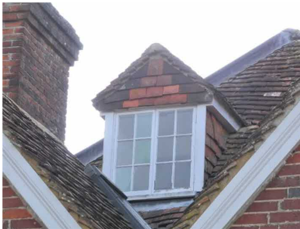
Figure 38: Exterior of window S1
