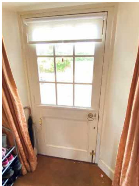
Figure 41: Interior view of the front door
