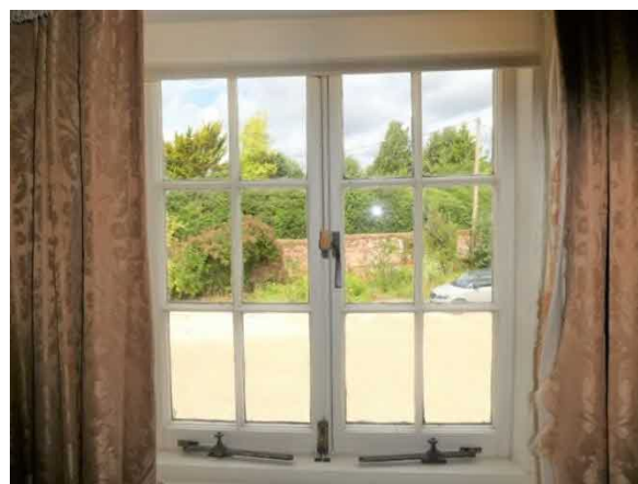
Figure 34: Interior view of window F3
