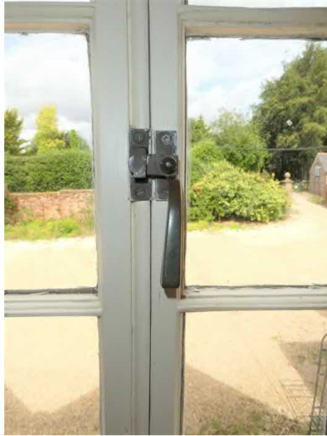
Figure 30: Detail of a bronze casement catch – window F1
