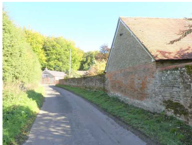
Figure 2: Boundary wall at Weston Corbett House
