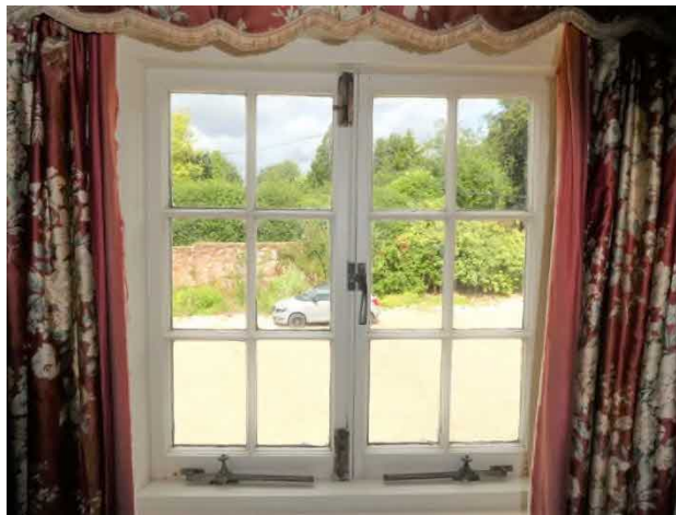
Figure 28: Internal view of window F1
