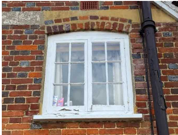
Figure 35: Exterior of window F4
