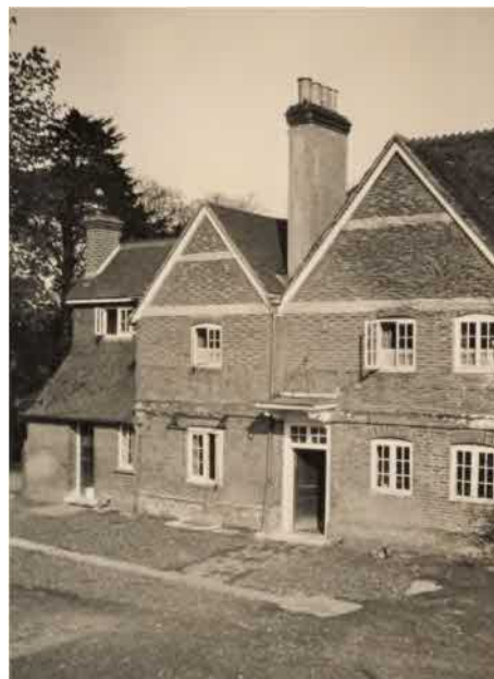
Figure 16: View of the left hand side of the north-west elevation of the house before the flat roof extension was added
