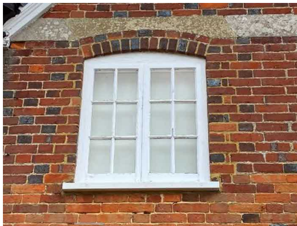
Figure 31: Exterior of window F2
