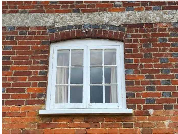
Figure 27: Exterior of window F1
