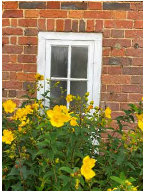
Figure 21: Exterior of window G3
