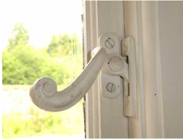
Figure 25: Detail of a G5 window fitting (catch)
