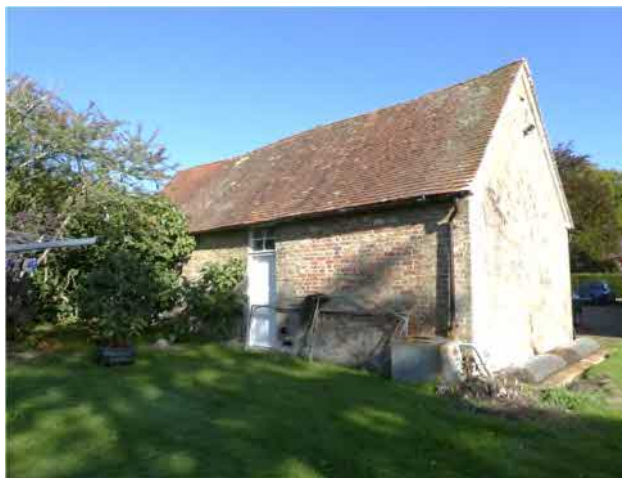
Figure 5: Garage at Weston Corbett
