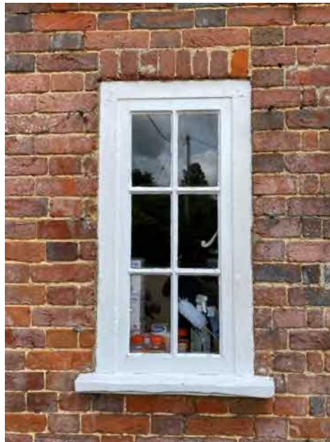
Figure 20: Exterior of window G1
