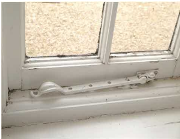
Figure 26: Detail of a G5 window fitting (stay)
