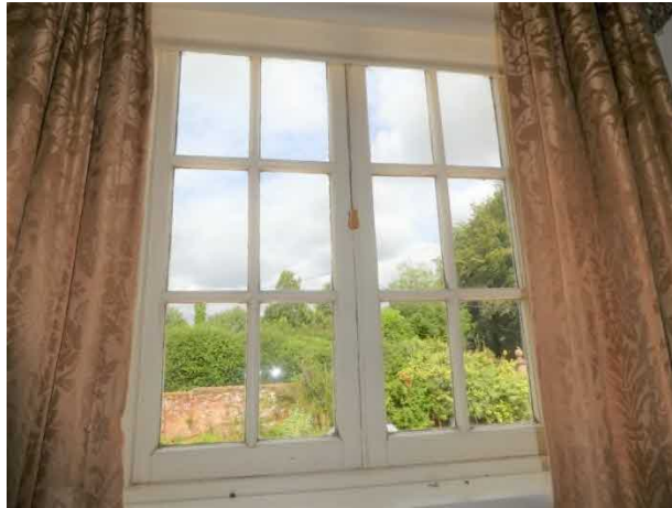
Figure 32: Interior view of window F2
