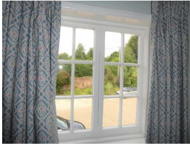
Figure 37: Interior view of window F5
