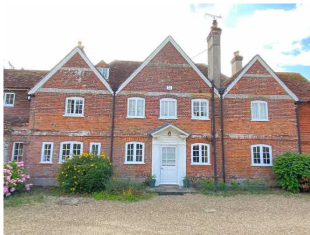
Figure 18: Central portion north-west elevation of Weston Corbett House
