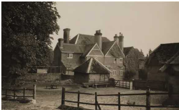
Figure 15: Photograph showing the rebuilt north-east extension before the flat roof elements were added
