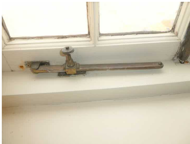
Figure 29: Detail of a brass telescope casement stay – window F1
