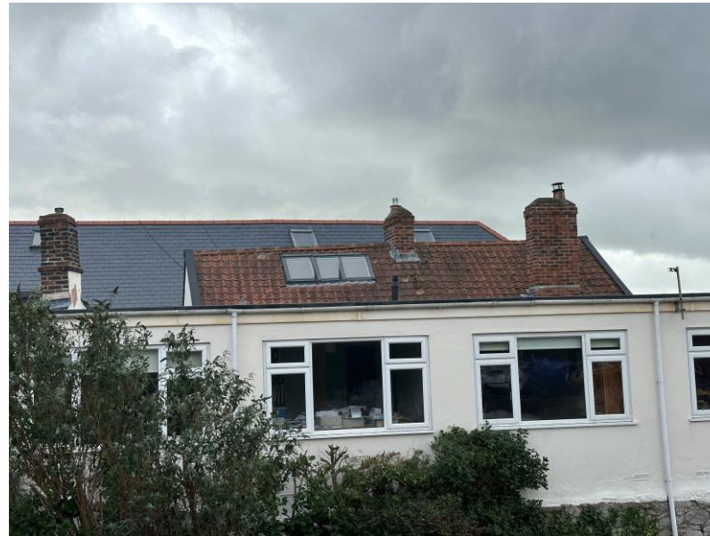
4. Replacement extended roof window – side view
