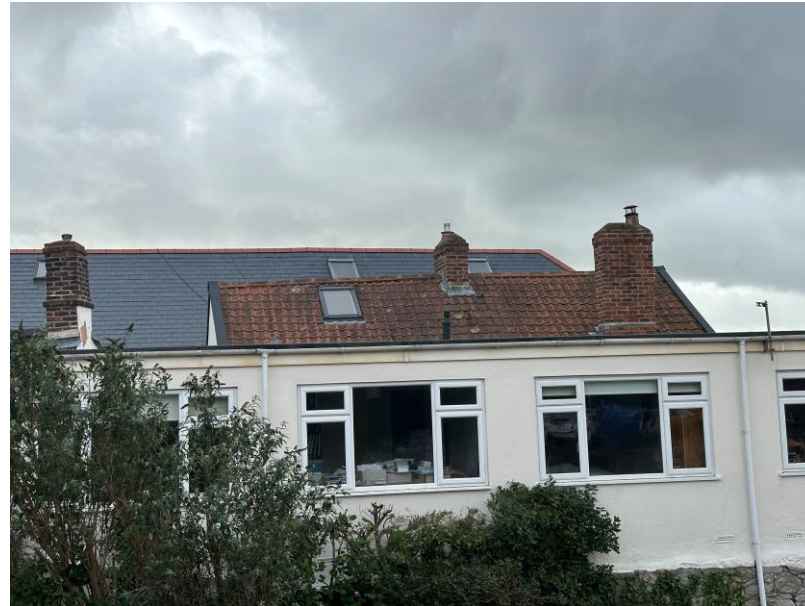
2. Existing roof window – side view
