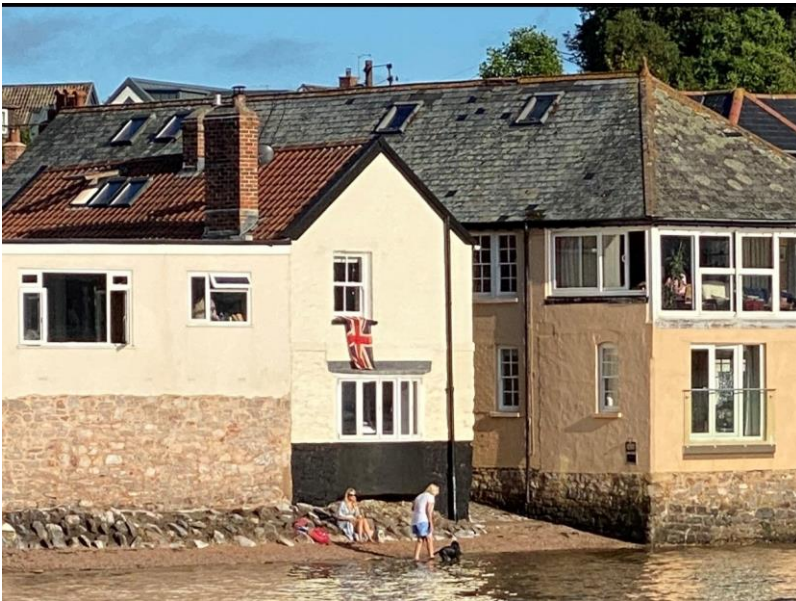
3. Replacement extended roof window – front view
