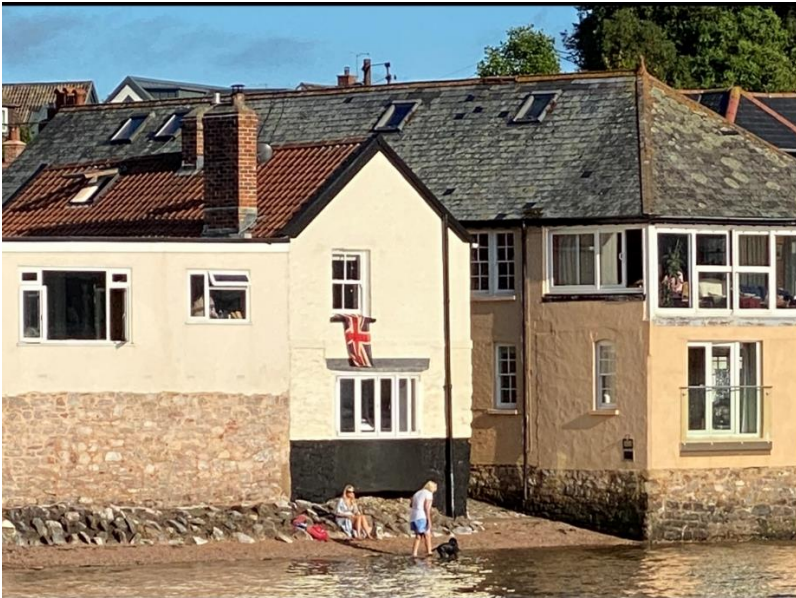
1. Existing roof window – front view
