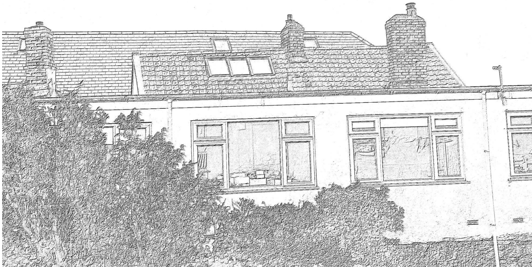
3. Replacement extended roof window – side view
