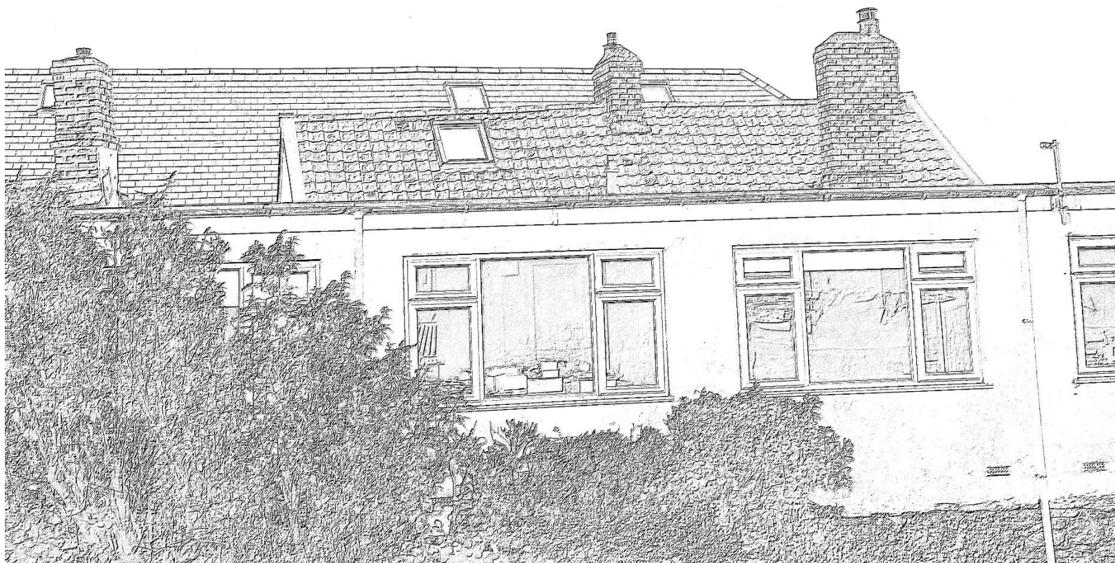
1. Existing roof window – side view
