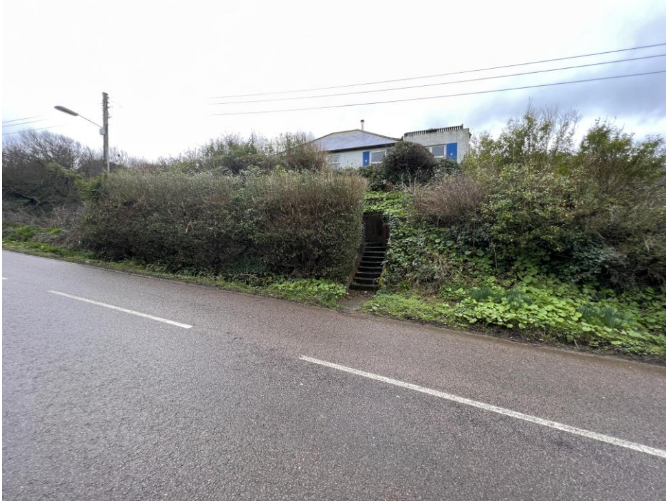
Photograph showing existing Sea Lodge from Tregurrian Hill
