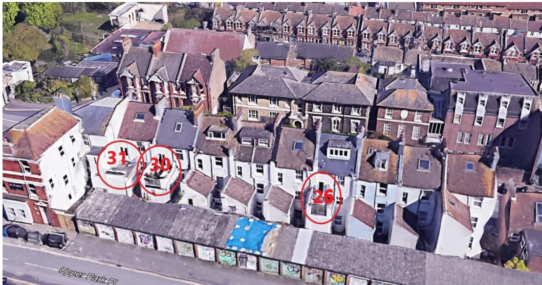
Figure 2: Terrace of west side of Egremont, northern end. Roof terraces at 26, 30 and 31
