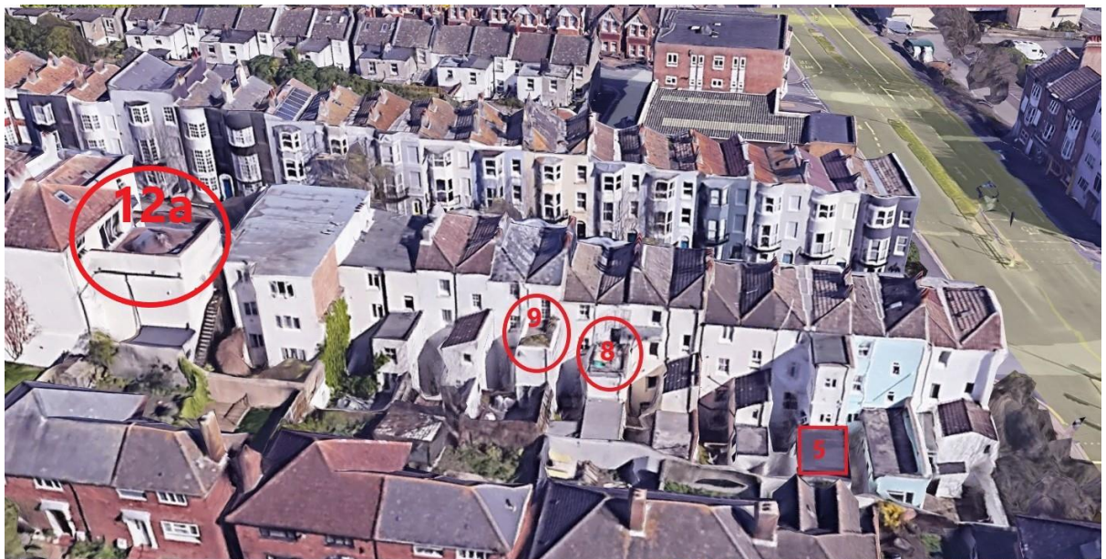
Figure 3: West side of Egremont Place, southern end. The application site is shown in the red square. Three further roof terraces, at 8, 9 and 12a Egremont Place, are visible.
