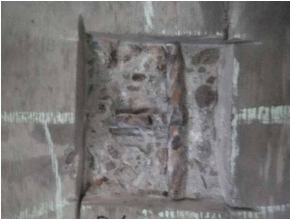
Plate 27 – Showing a close up view of breakout B/O8.
