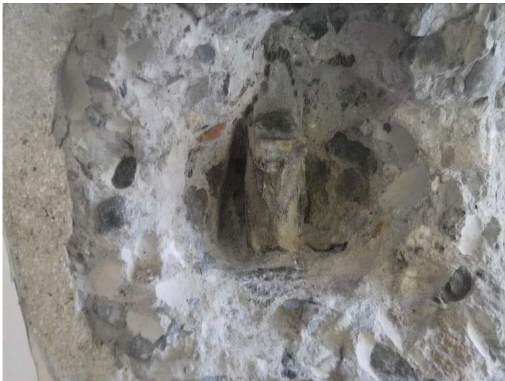
Plate 16 – Showing a close up view of breakout B/O2.
