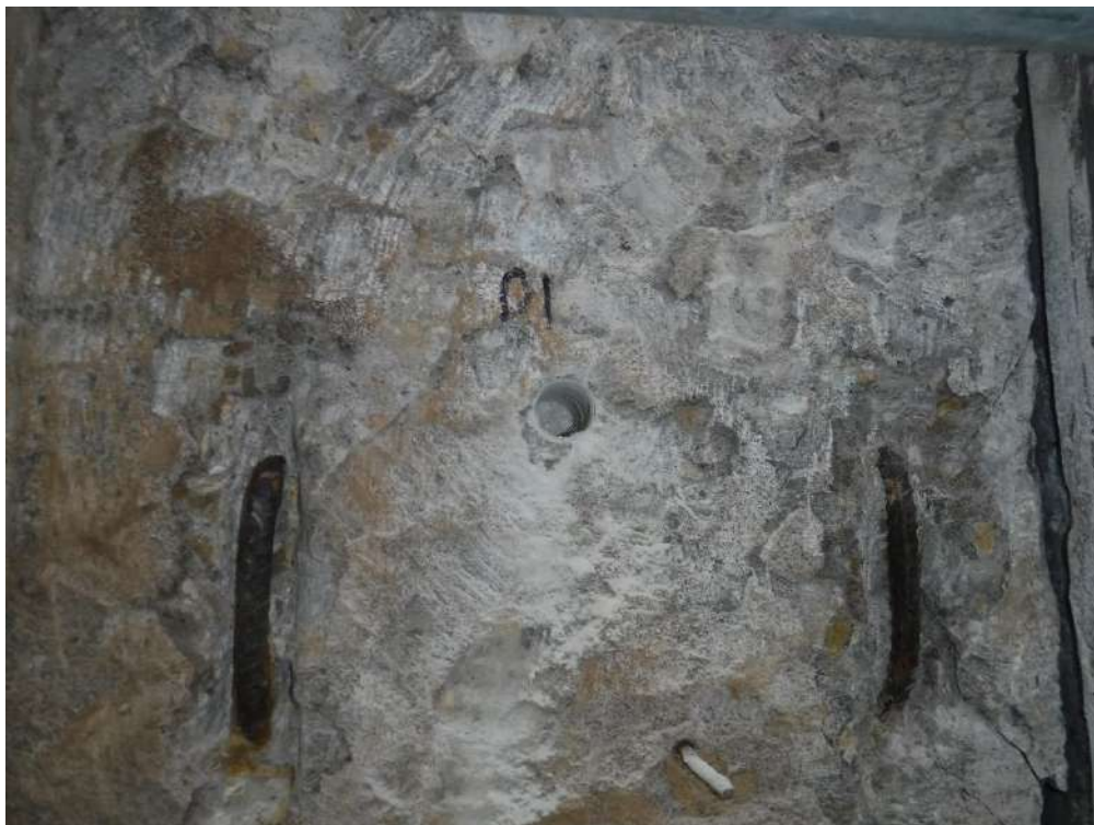
Plate 10 – Showing a close up shot of drill hole D1 on lower panel breakout
