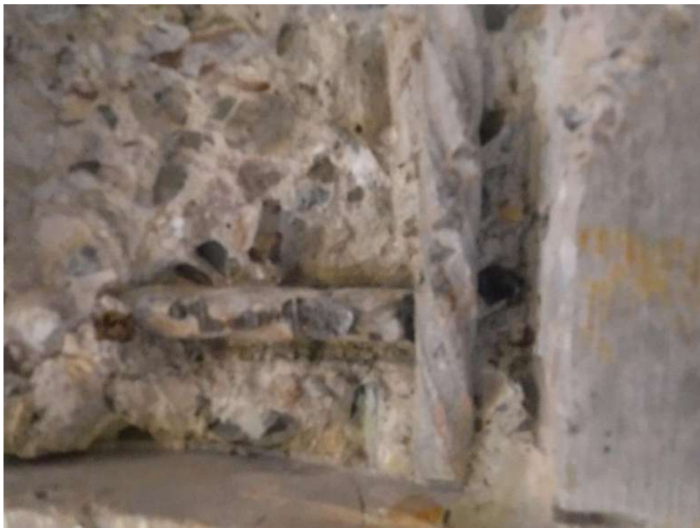
Plate 18 – Showing a close up view of breakout B/O3.
