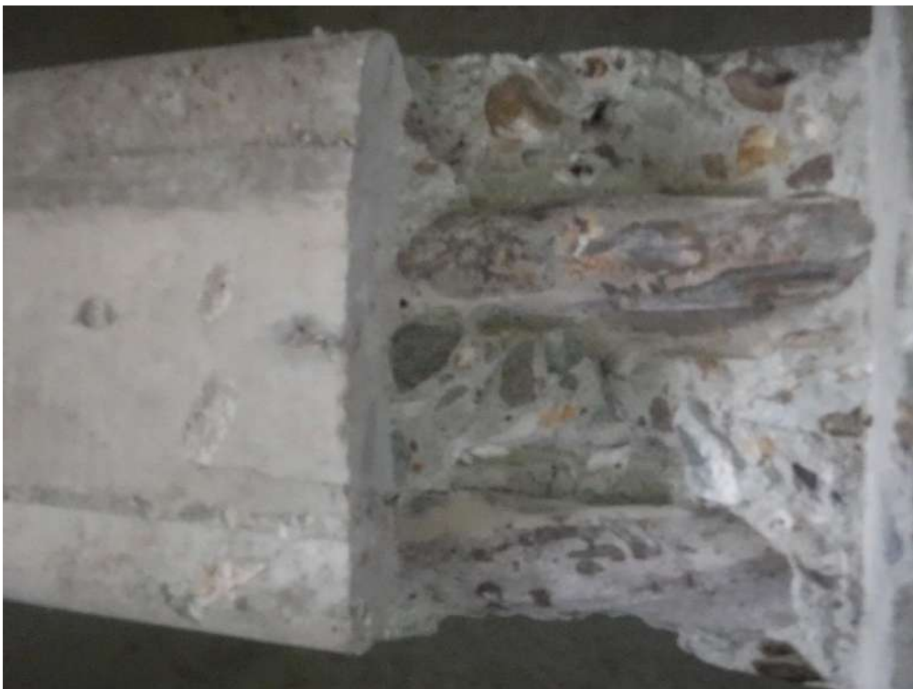
Plate 20 – Showing a close up view of breakout B/O5.
