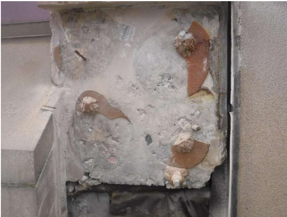
Plate 7 – General Shot of Top right-hand side panel breakout.
