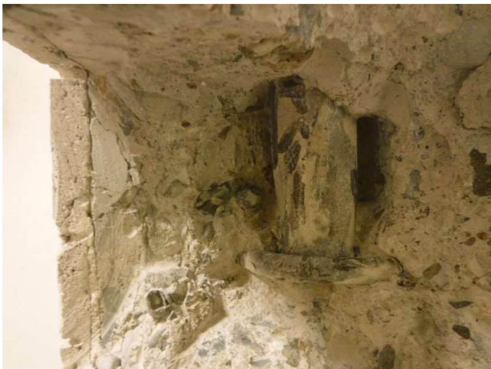
Plate 24 – Showing a close up view of breakout B/O7.
