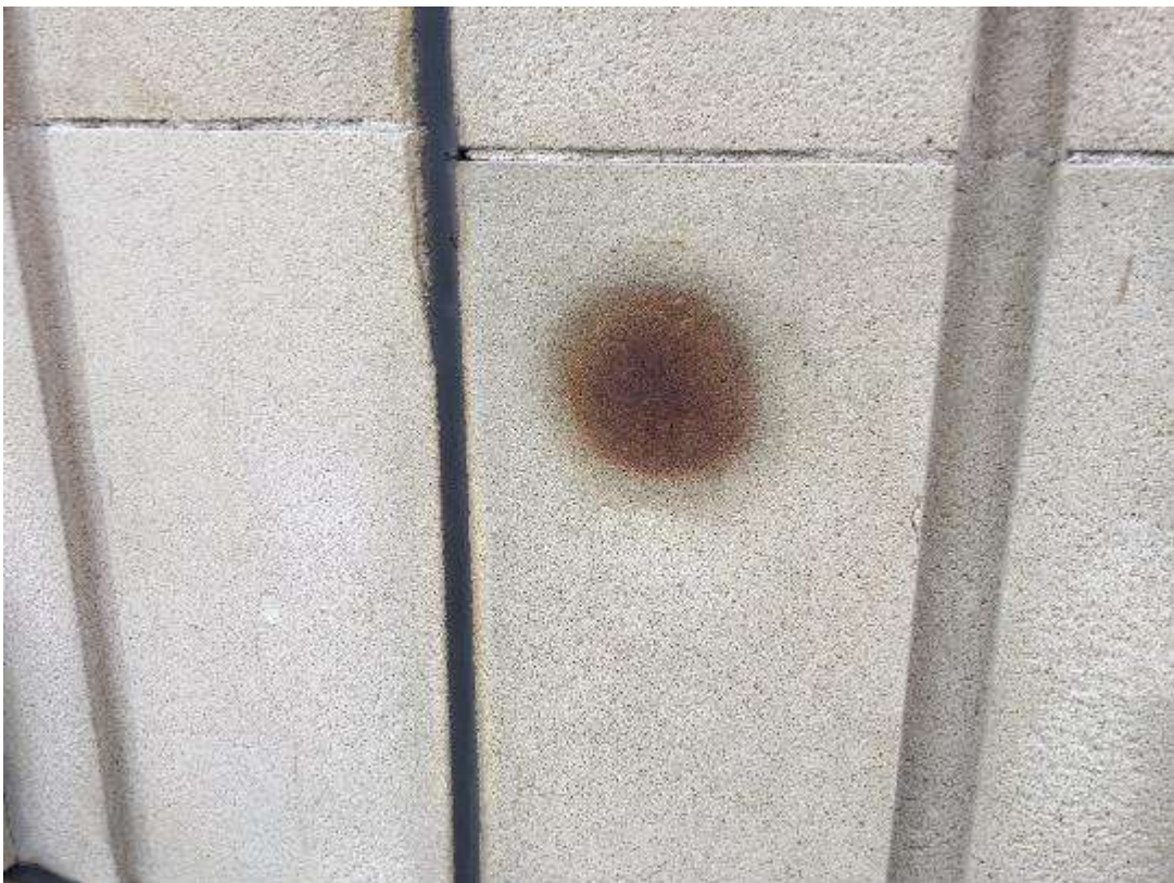
Photograph 2 Example of local discolouring
