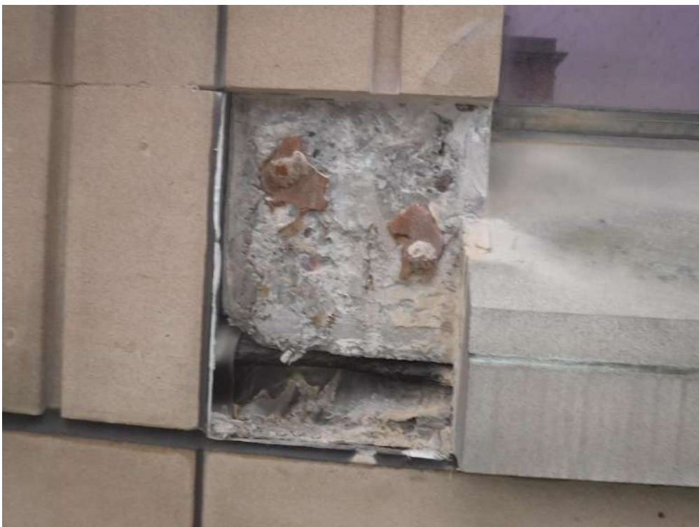
Plate 8 – General Shot of Top left-hand side panel breakout.
