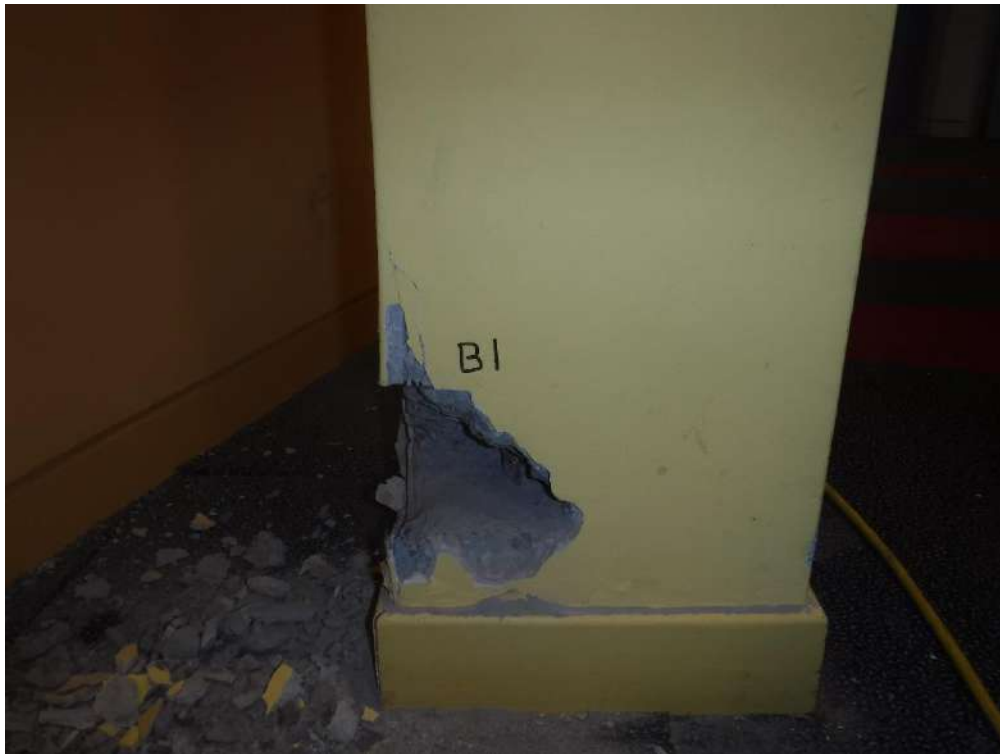
Plate 13 – Showing a general view of breakout B/O1 (internal column 1 st floor).
