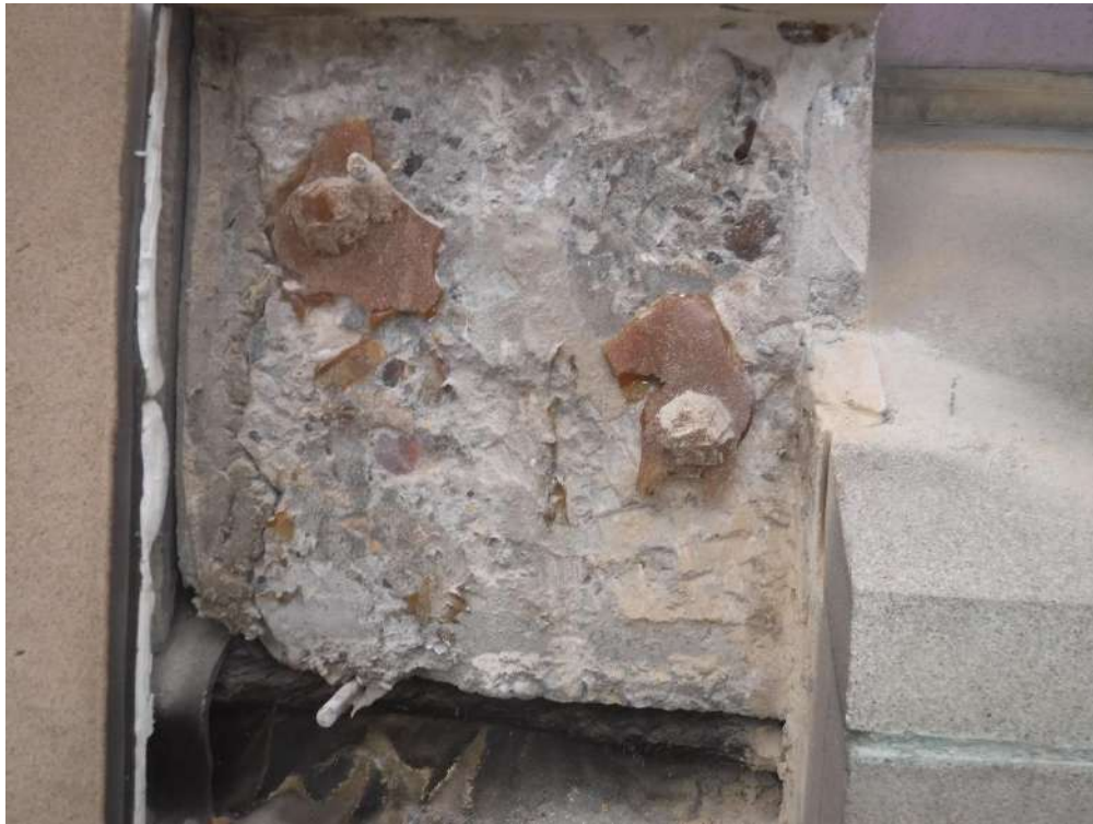
Plate 9 – Close up Shot of Top left-hand side panel breakout.
