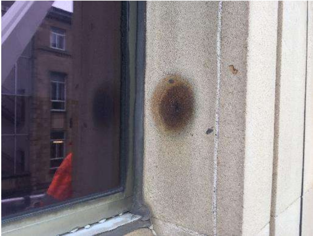
Photograph 1 Example of local discolouring
