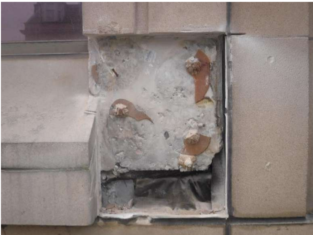
Plate 6 – General Shot of Top right-hand side panel breakout.
