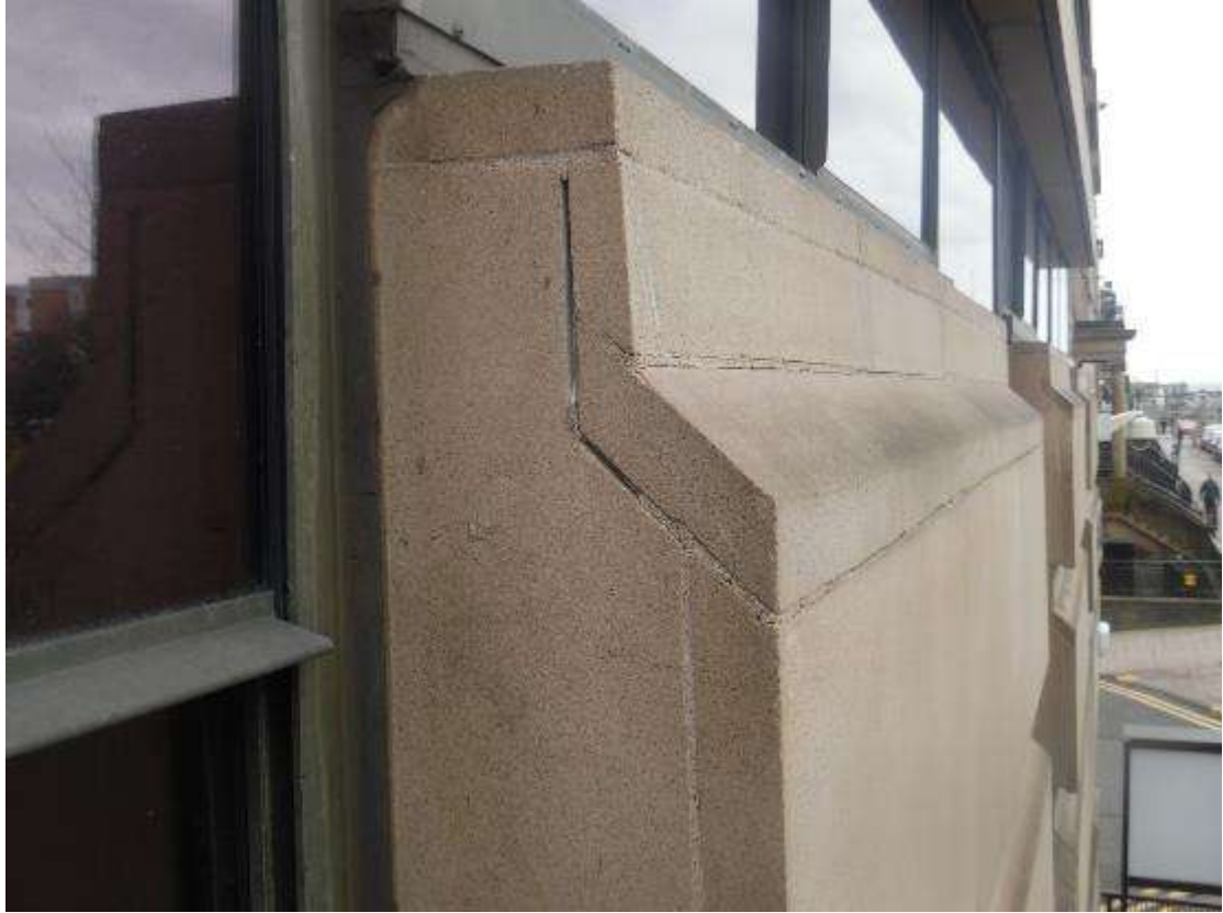
Photograph 10 Pointing on panel 3/9
