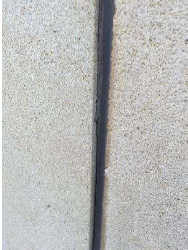
Photograph 6 - Mastic Seal Broken (Panel 4/7, Blytheswood Street elevation)
