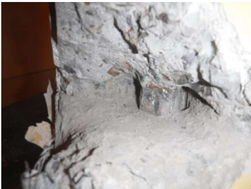
Plate 14 – Showing a close up view of breakout B/O1.
