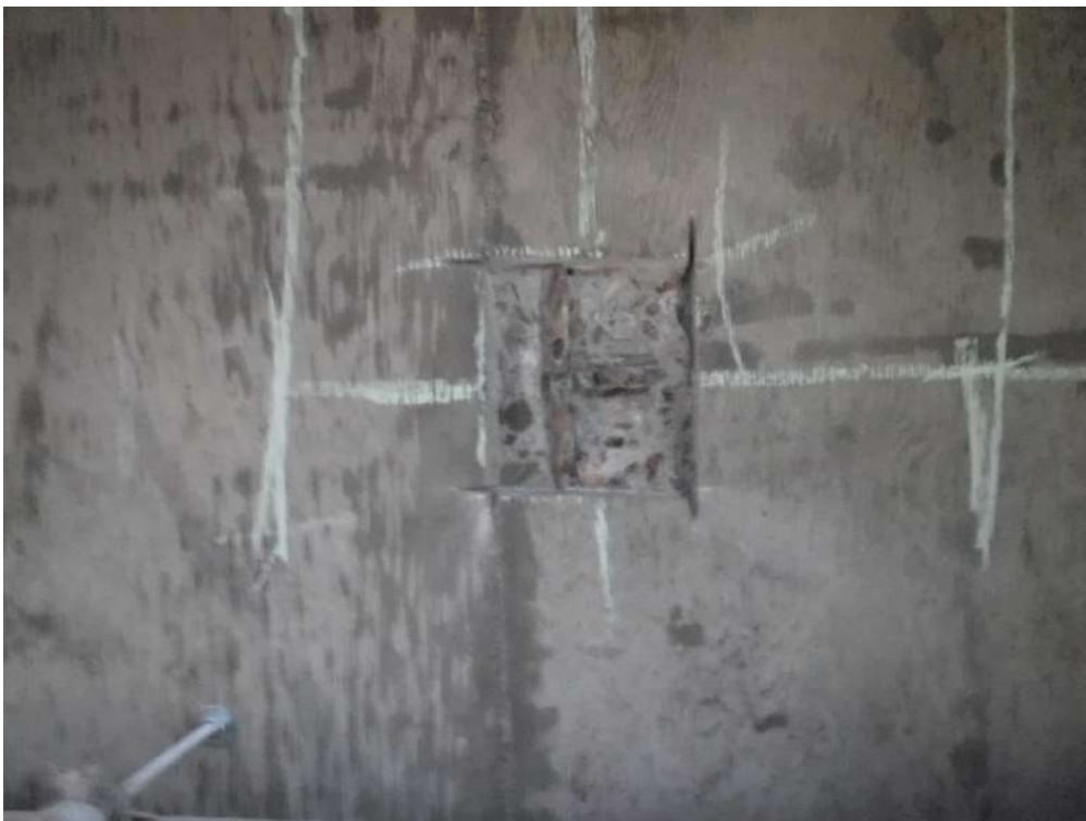
Plate 26 – Showing a general view of breakout B/O8 (underside of roof slab).
