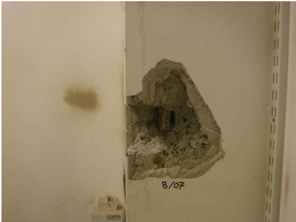
Plate 23 – Showing a general view of breakout B/O7 (5 th floor internal column).
