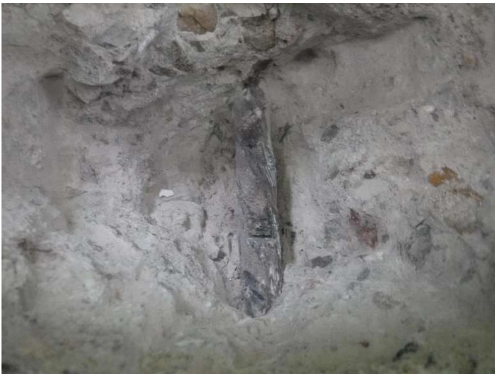
Plate 22 – Showing a close up view of breakout B/O6.
