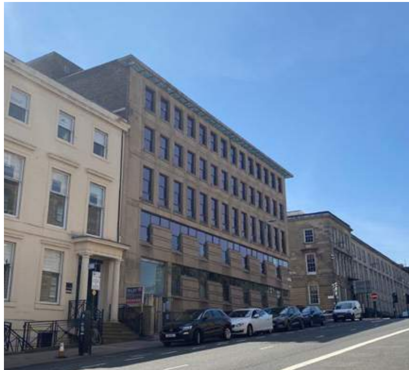
View from West George Street
