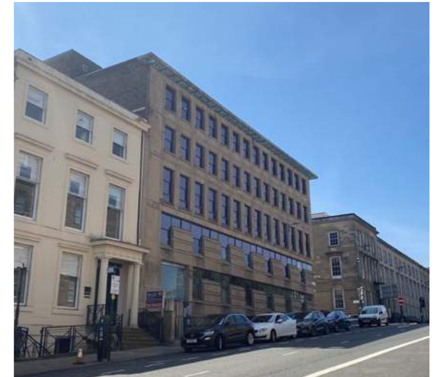
View from West George Street
