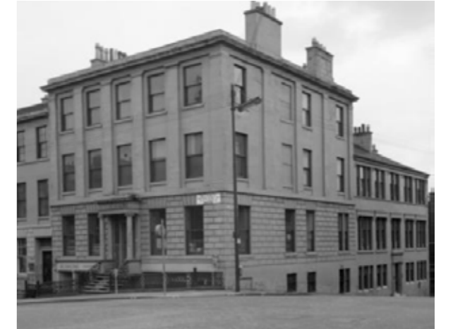
Original building on site (pre 1973)
