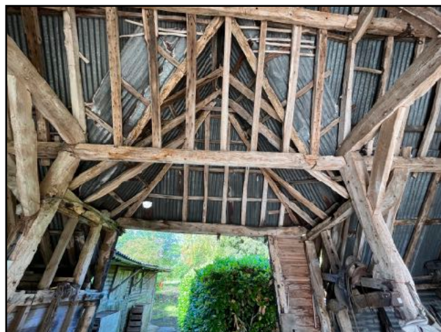
Image 12: Internal aspect (facing west) of B2
