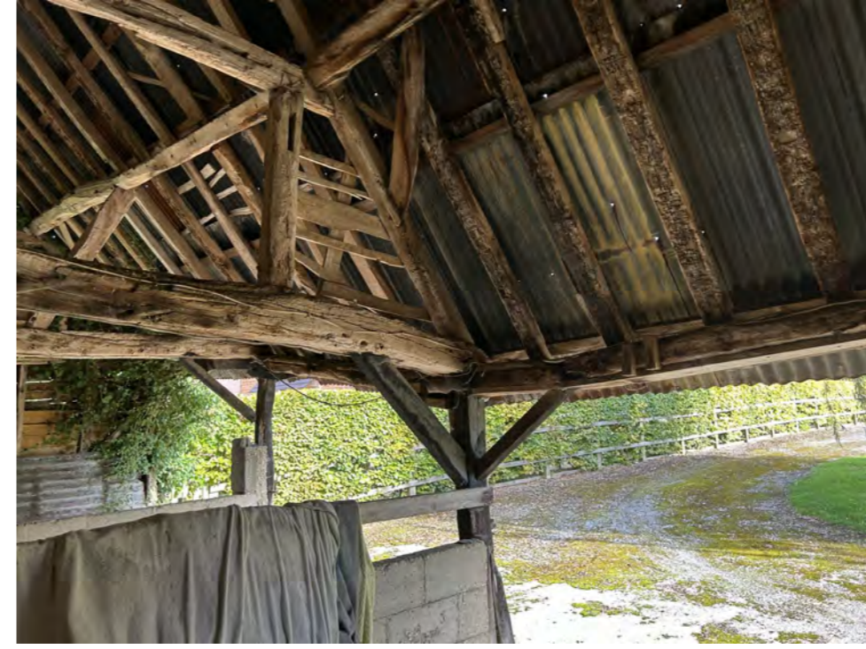
Bay adjacent to Threshing barn showing truss A
