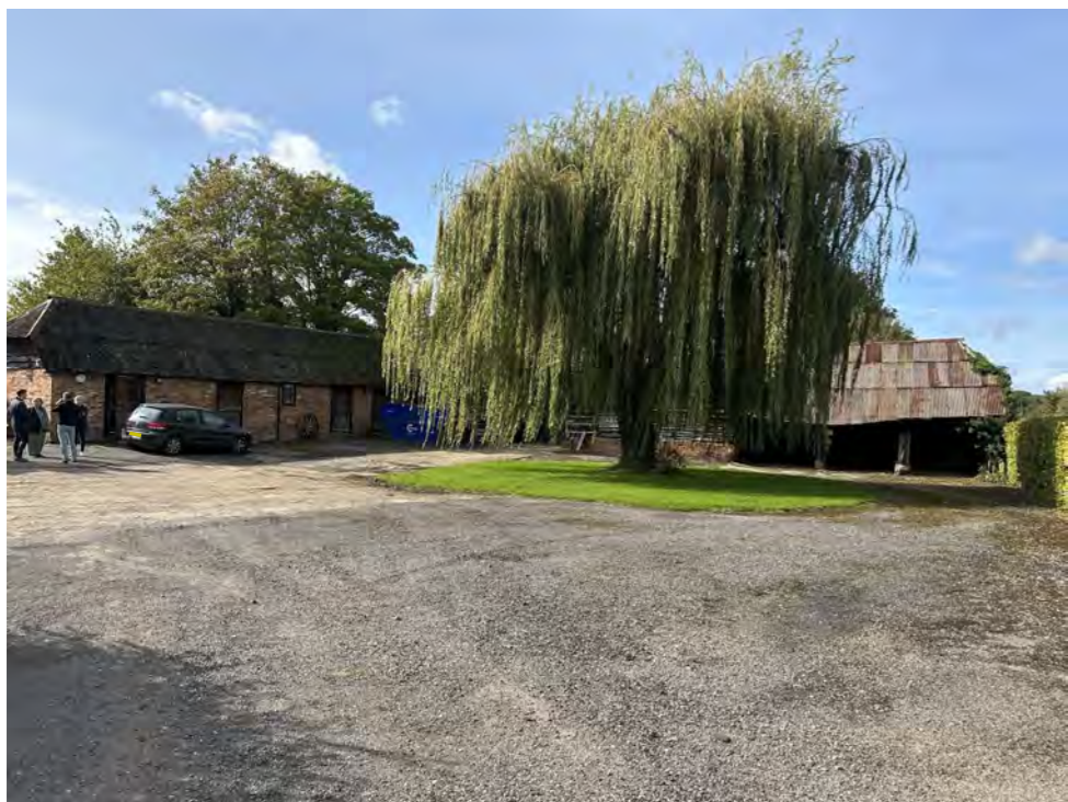
Courtyard to Barns
