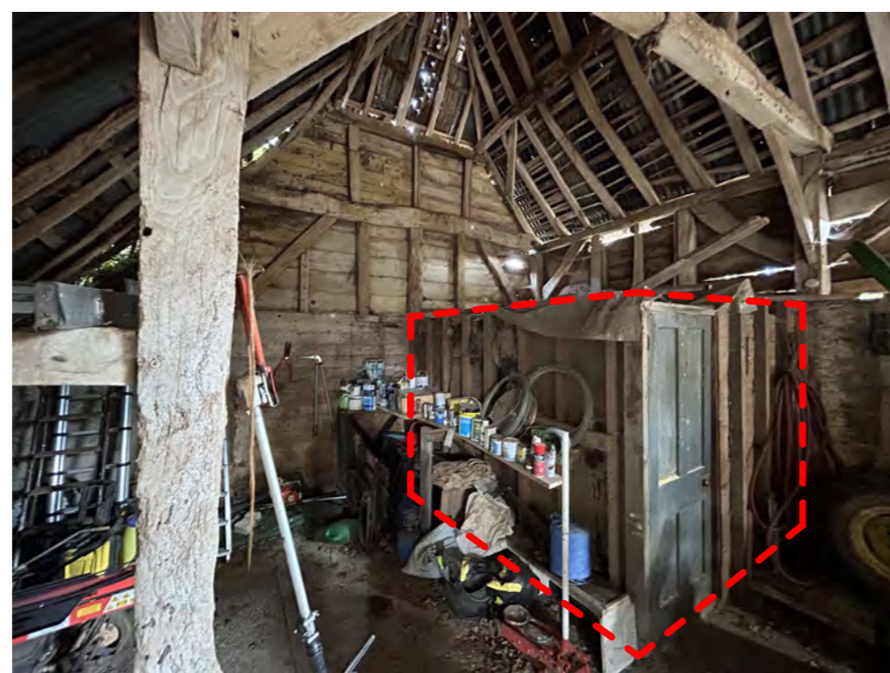
Existing Internal of Barn
