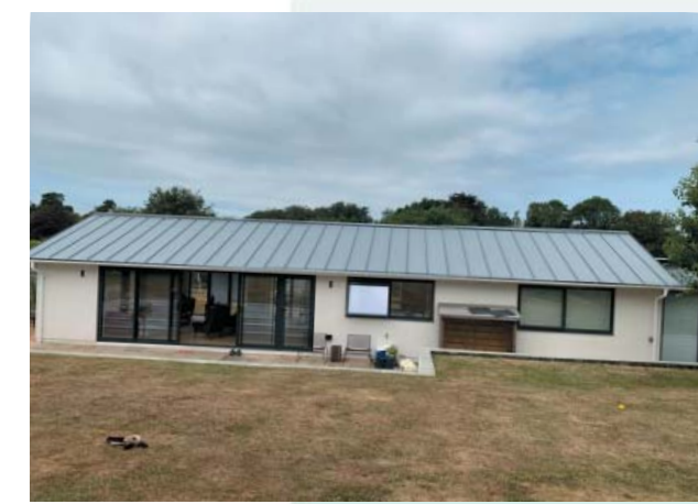
Rear view of south east elevation
