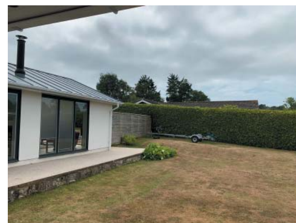
View looking south at boundary condition
