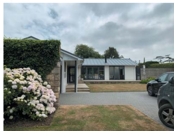
View looking south east into front elevation
