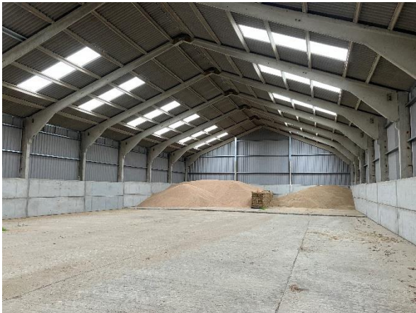
Photo 3: Internal view of Building 1
