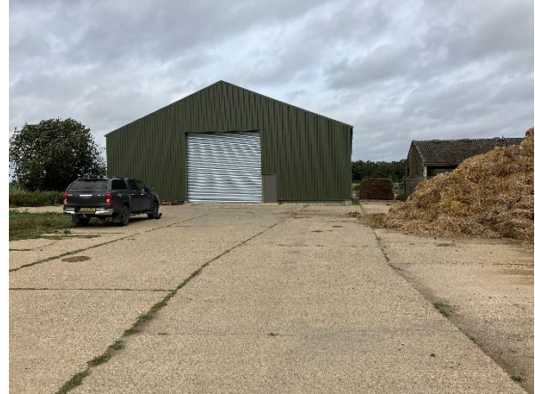
Photo 2: Southern façade of Building 1, and existing hard standing entrance to site
