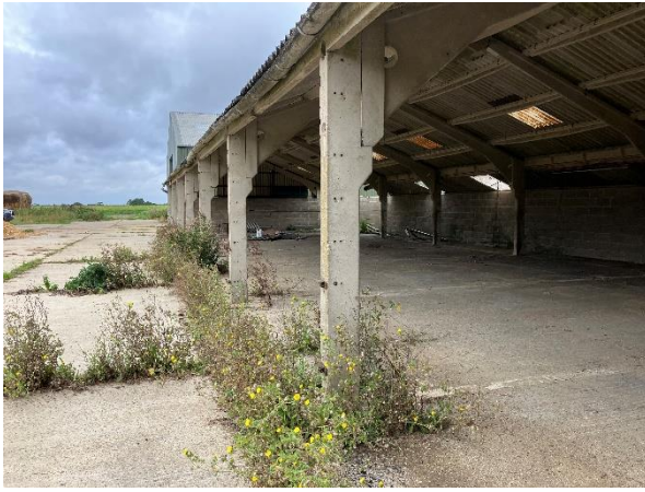
Photo 7: Structure of Building 2 – concrete supports and corrugated fibreboard sheets
