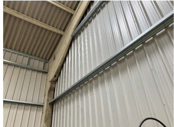
Photo 4: Wall structure of Building 1 – concrete and metal supports and walls
