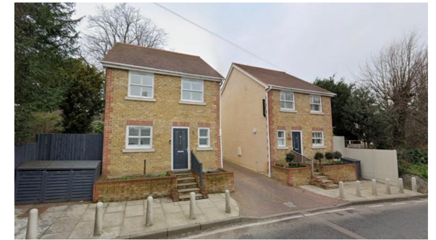
52 Baston Road viewed from the road in front.
