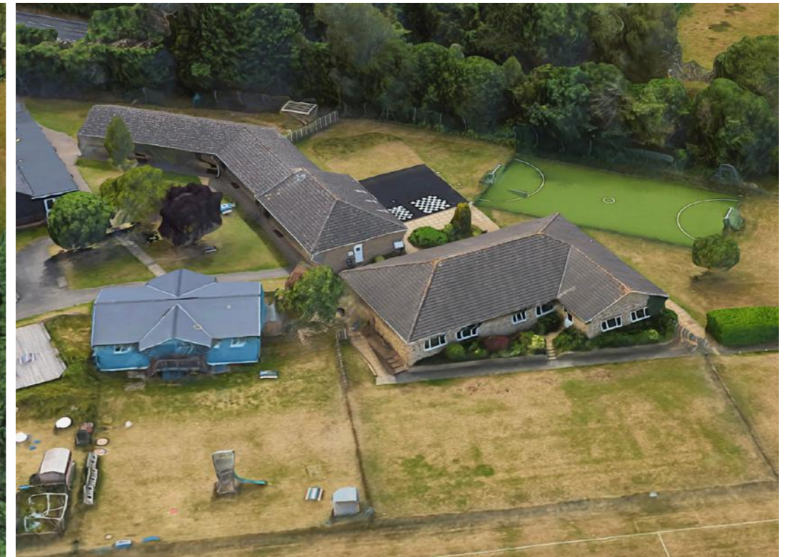
Cluster of school buildings to the south of the site, sat within the green belt
