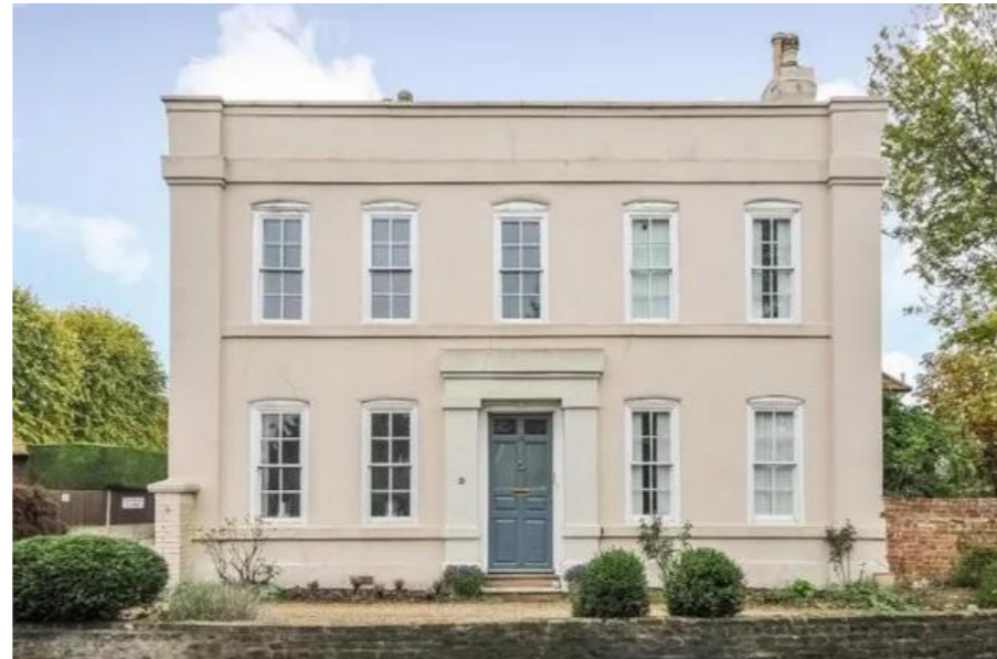
Ash Lodge, opposite the site entrance
