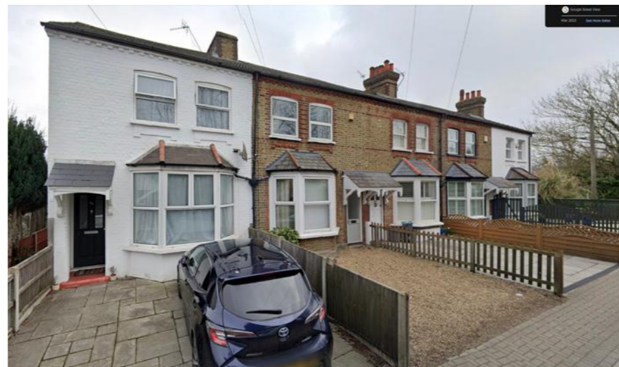
Bath Villas, 121-131 Baston Road
