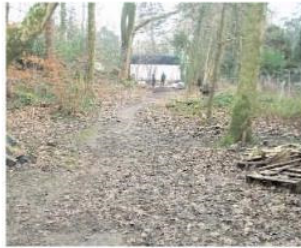
Access road for the National Lake District Parks Authority. Site before construction pictured above.
