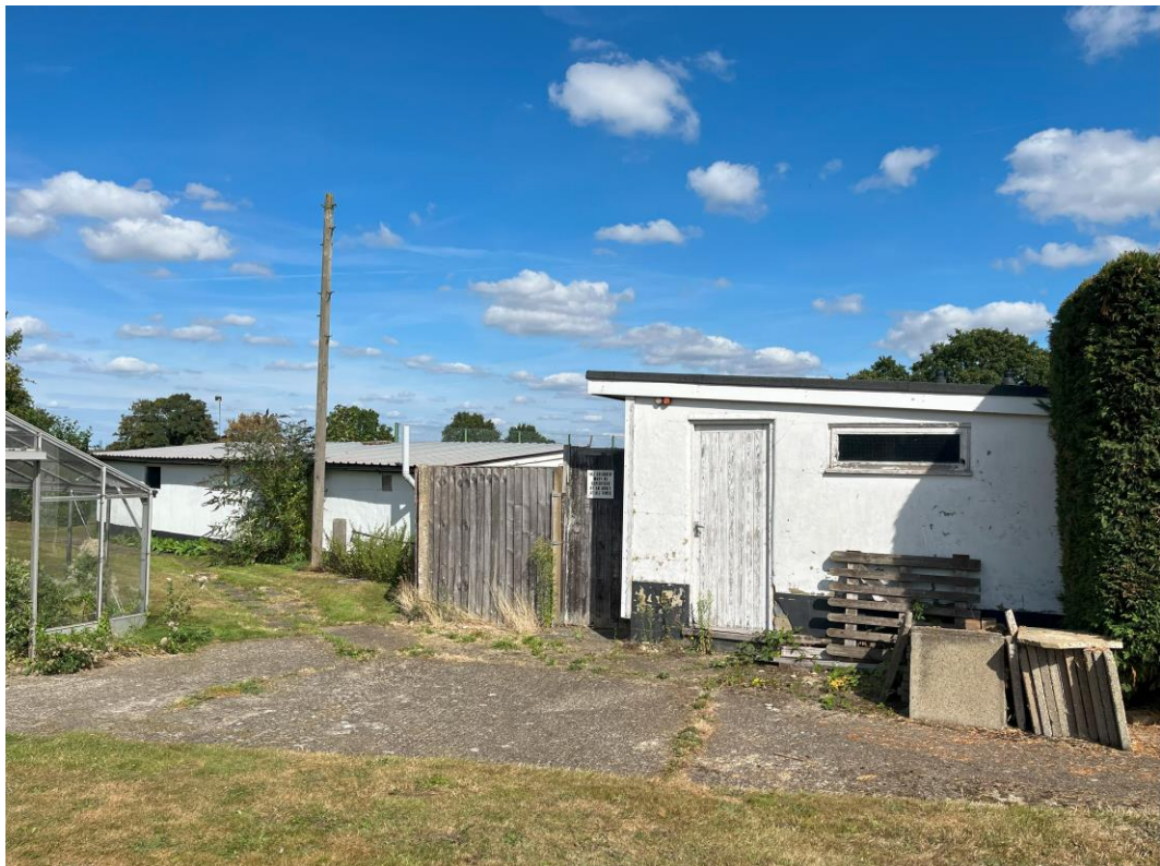
Figure 13: Built form associated with the former swimming pool and sports court
