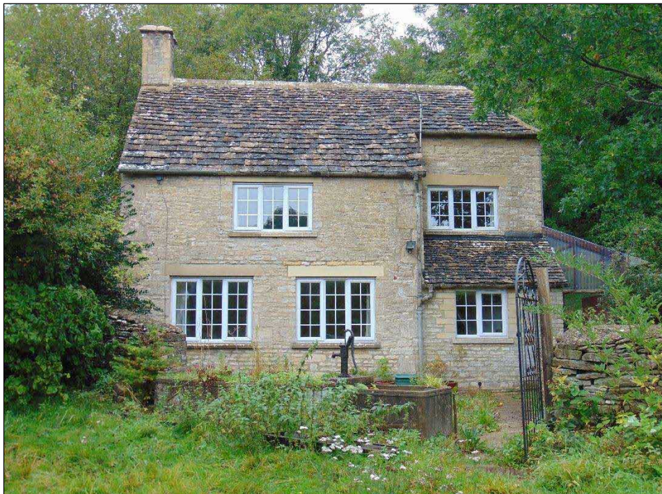
Above: western elevation of the cottage
