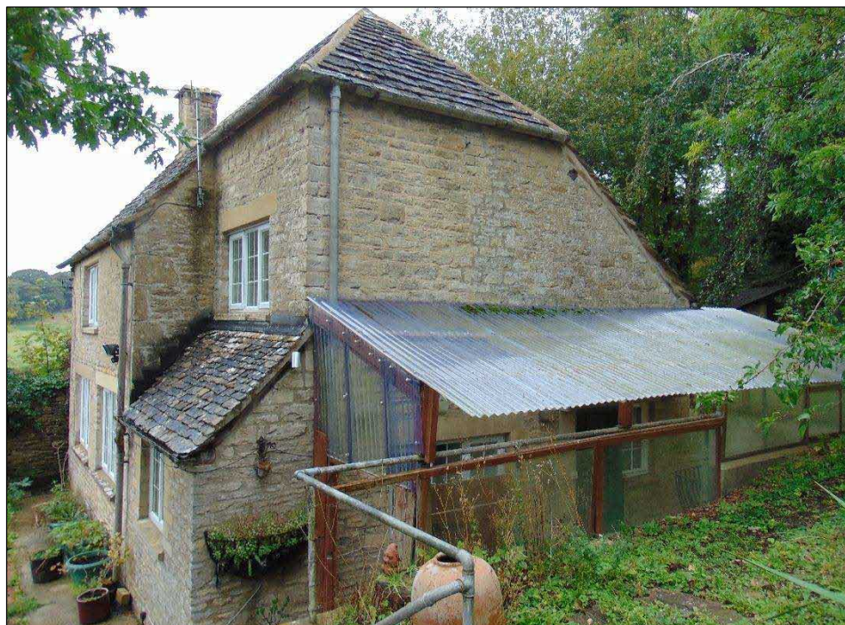
Above: the southern and western elevations of the cottage
