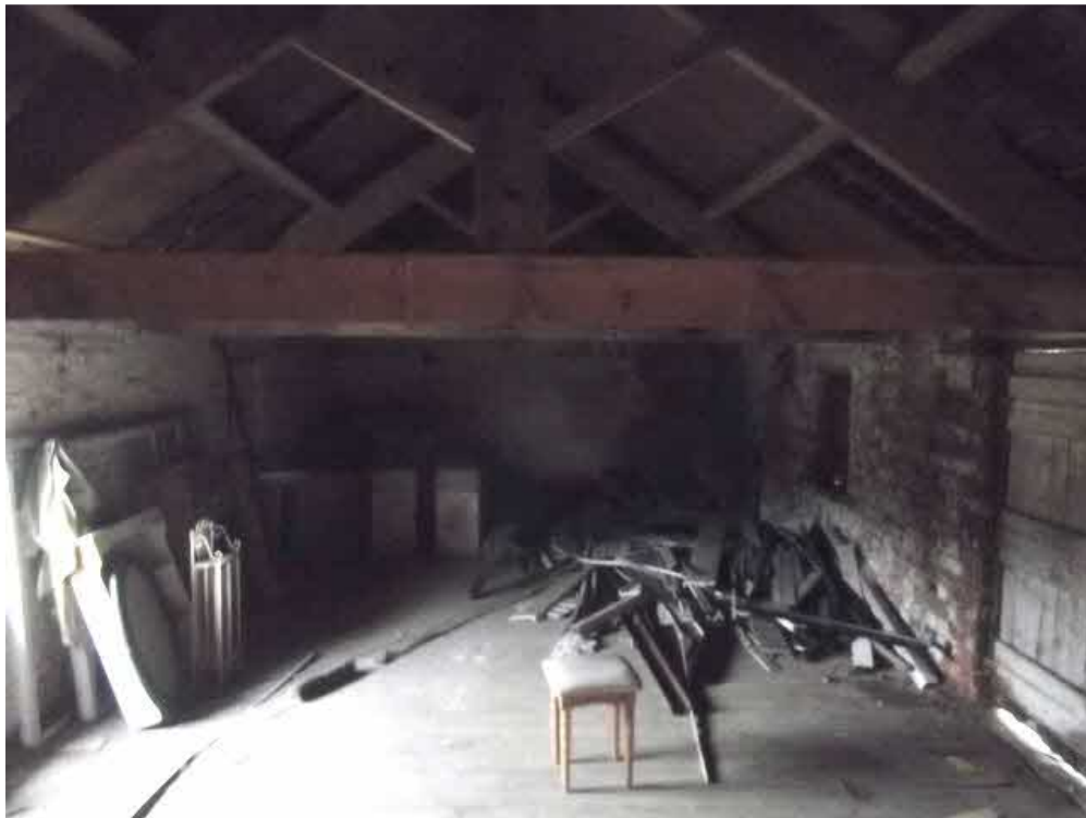
Plate 5. Interior of the first-floor level.
