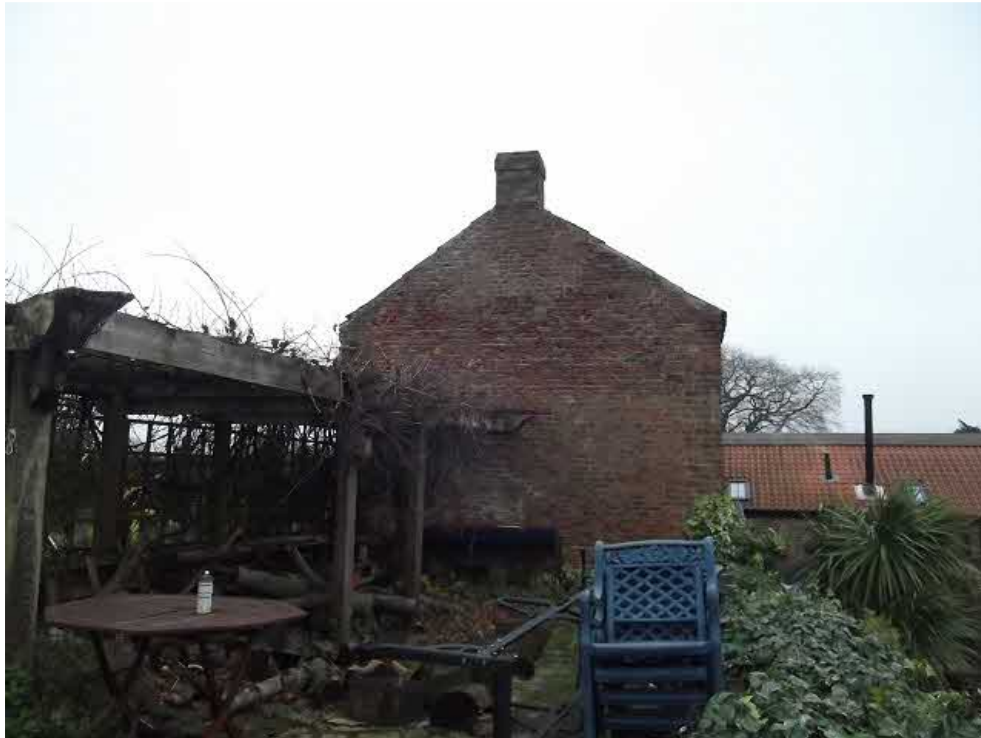
Plate 3. The northwest gable of the barn.
