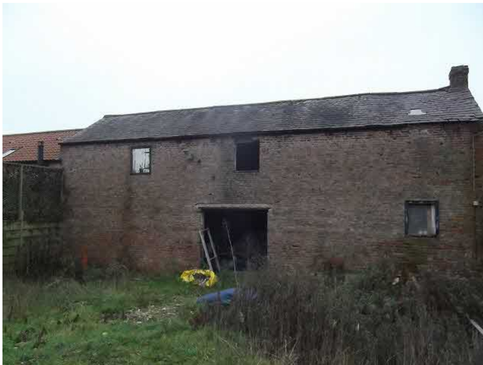
Plate 2. The northeast elevation of the barn.
