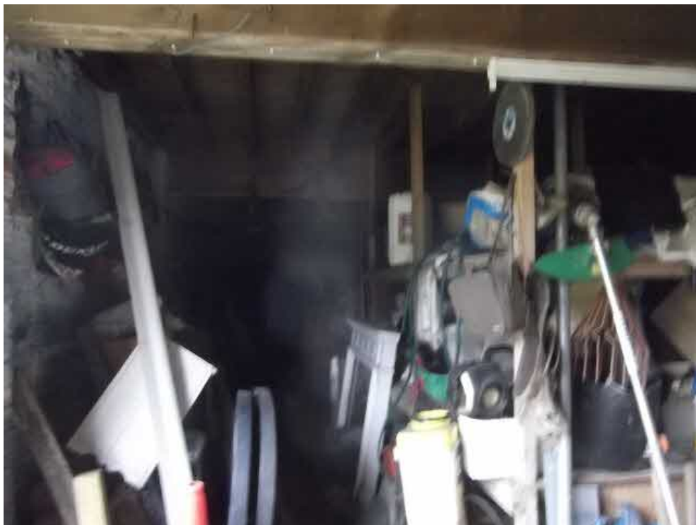
Plate 4. The interior of the ground floor.
