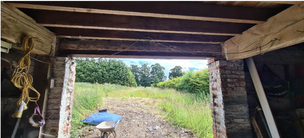
Pic 7 – Brick Pier to the rear
