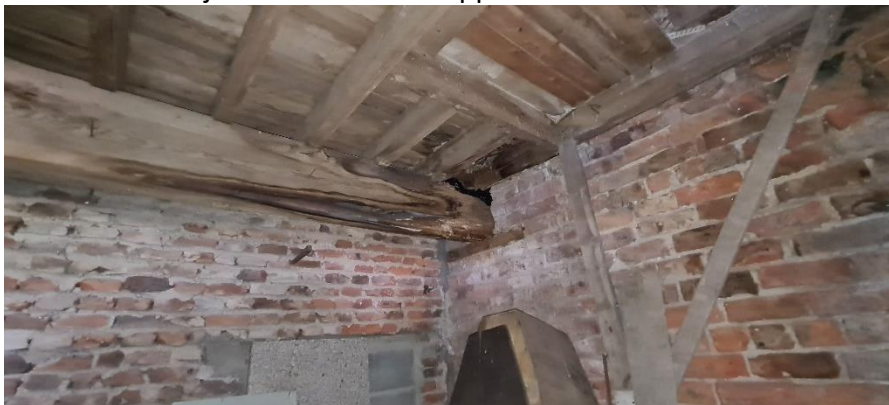
Pic 5 – 1 st floor joists and timber support
