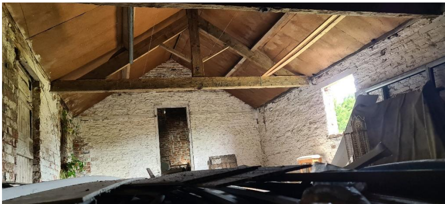
Pic 9 – External walls and trusses
