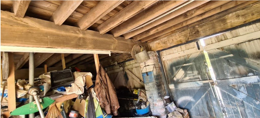
Pic 6 – Timber supports towards the front of the barn
