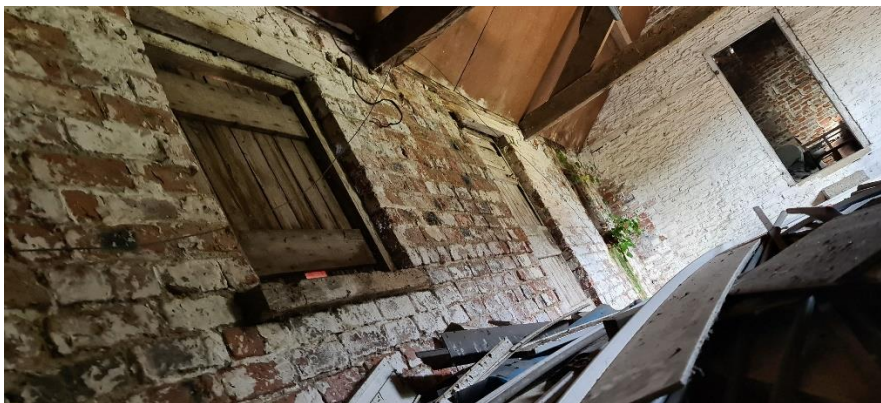
Pic 10 – Window to the front elevation
