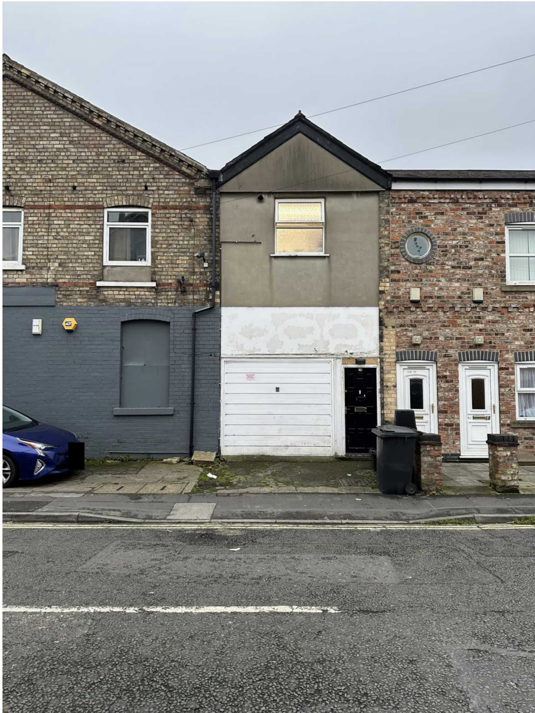
Front Elevation Facing Vyner Street
