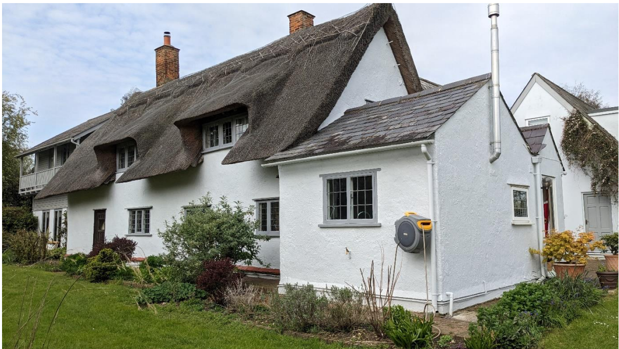
Photo 2: The cottage extension
