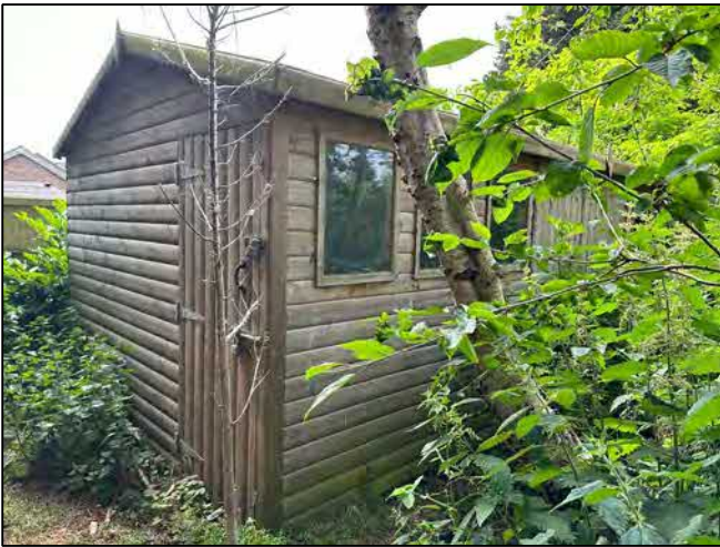
b) Timber shed on southern boundary.
