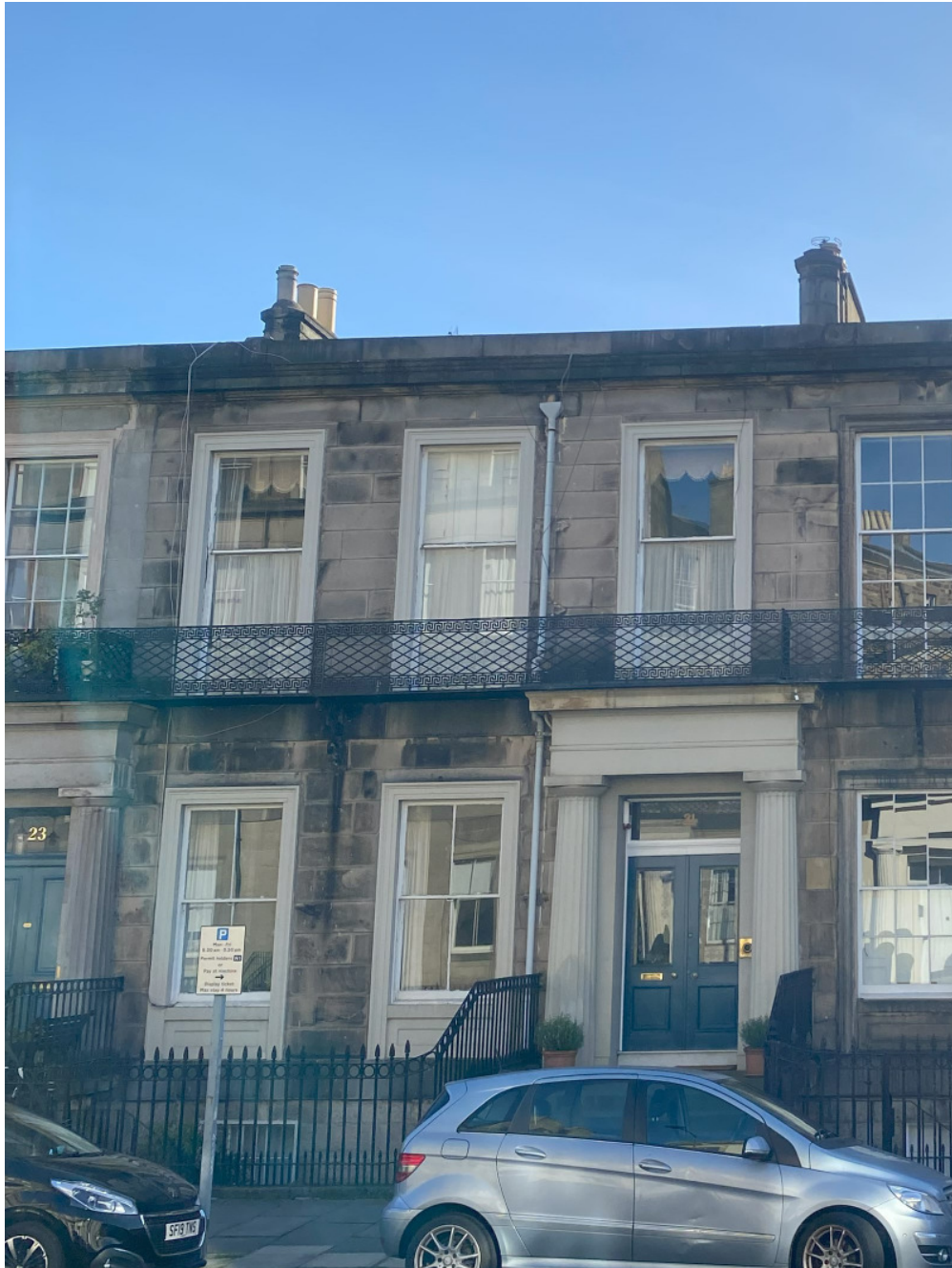
21 Windsor Street – Entrance Columns & Window Reveals Painted
