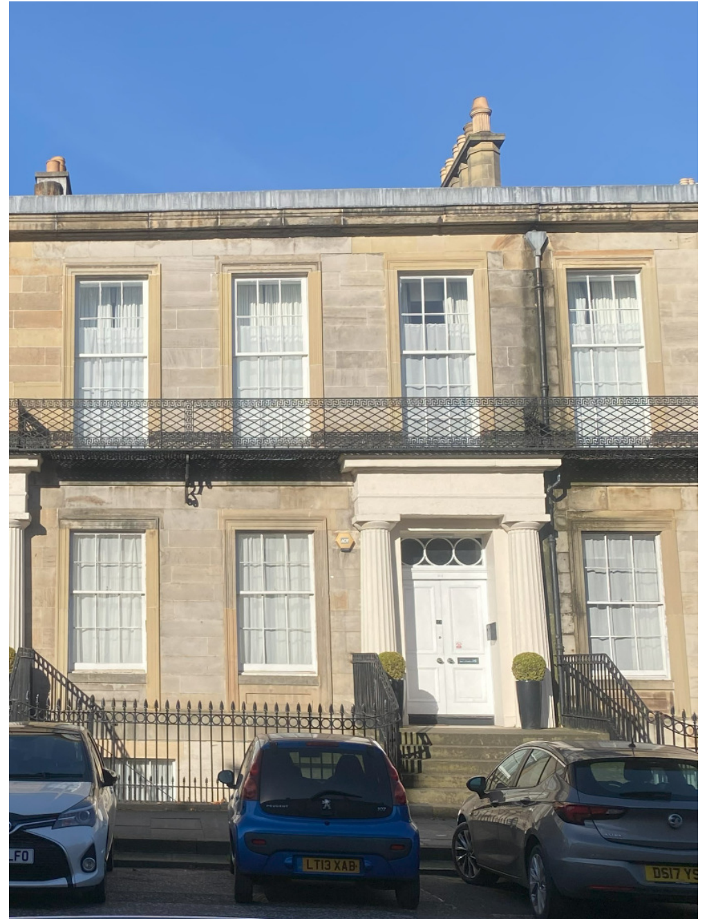
22 Windsor Street – Entrance Columns Painted
