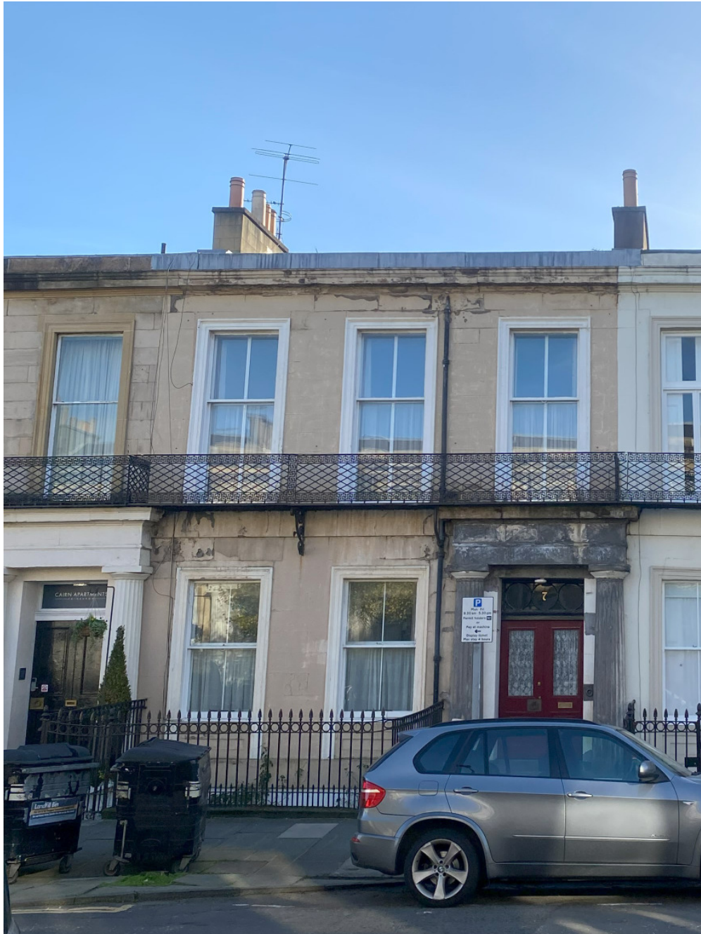
7 Windsor Street – Basement Wall Painted & Window Reveals Painted
