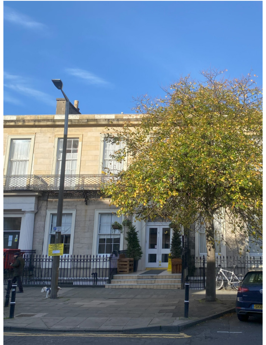
12 Windsor Street – Basement Wall, Entrance Columns & Window Reveals Painted
