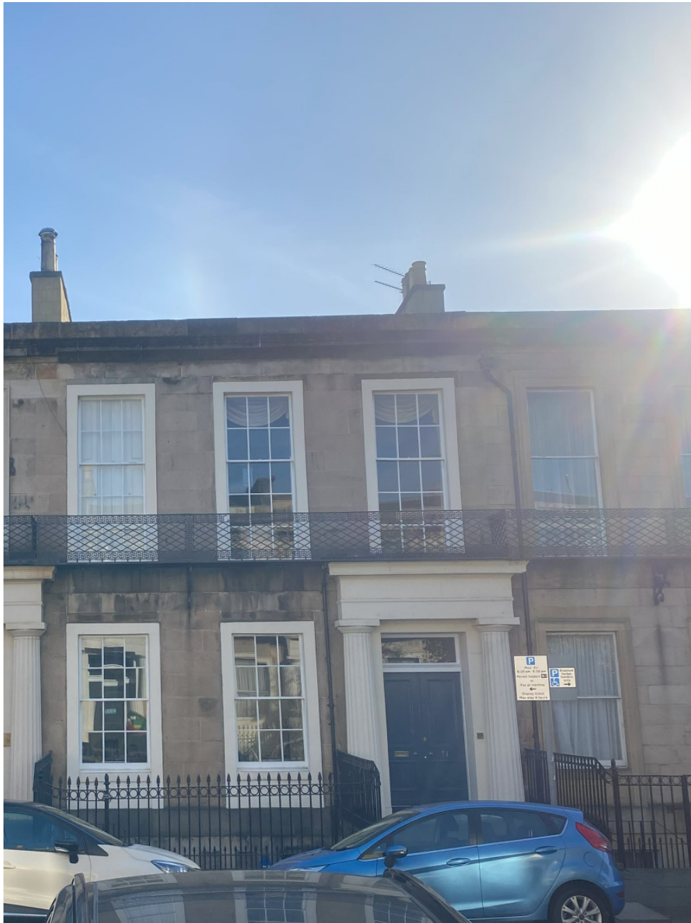
11 Windsor Street – Entrance Columns & Window Reveals Painted
