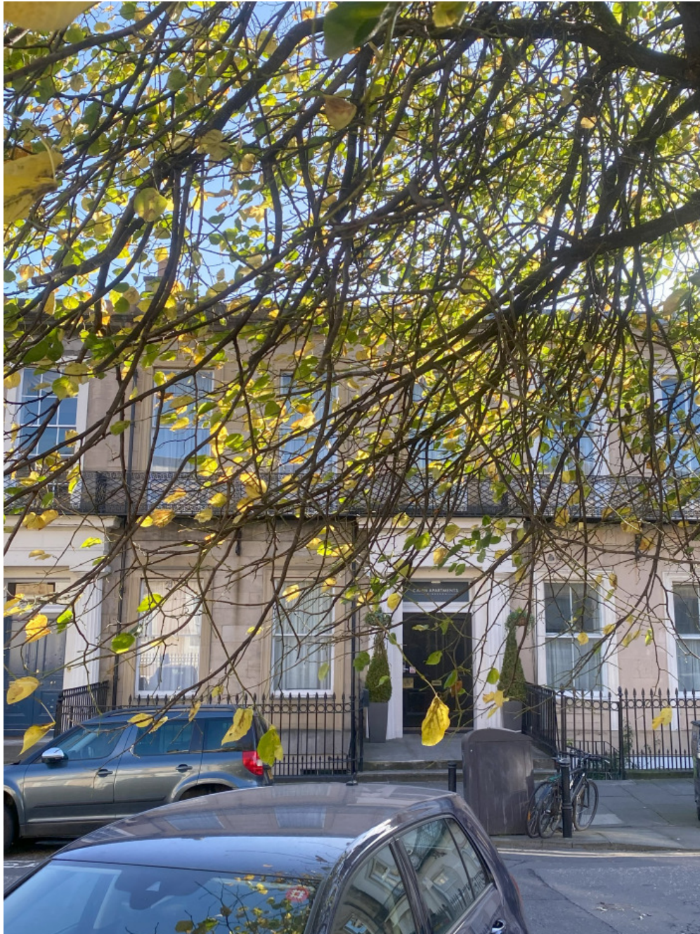
9 Windsor Street – Entrance Columns Painted
