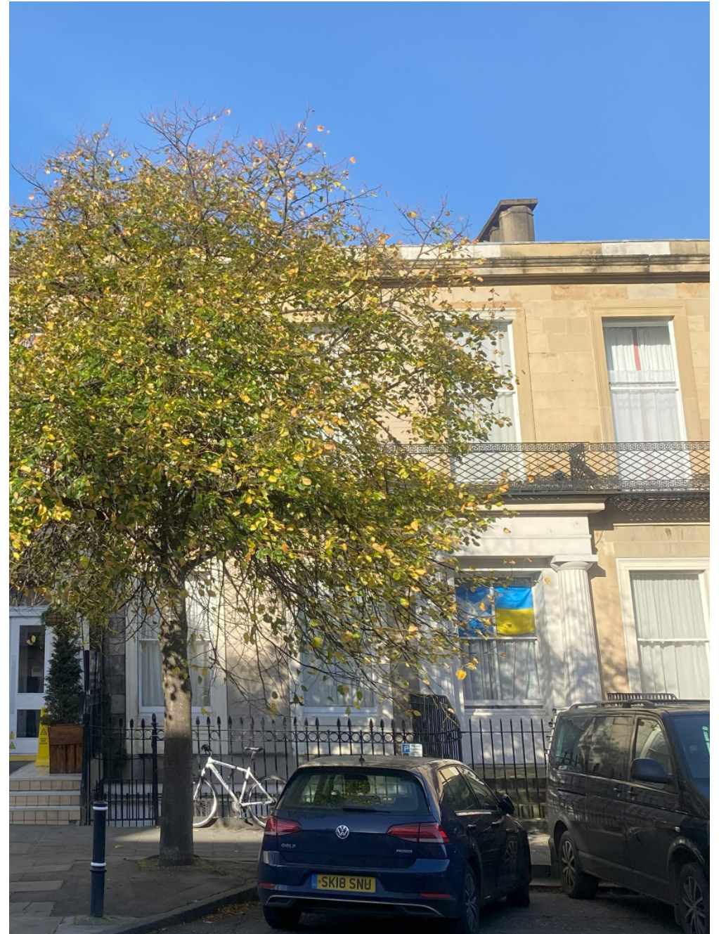
14 Windsor Street – Basement Wall, Entrance Columns & Window Reveals Painted
