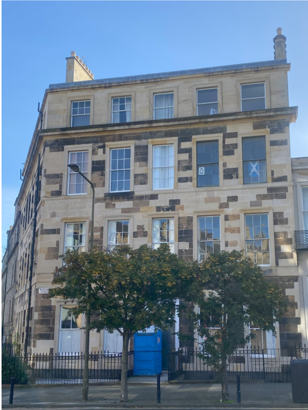
31 Windsor Street – Basement Wall Painted
