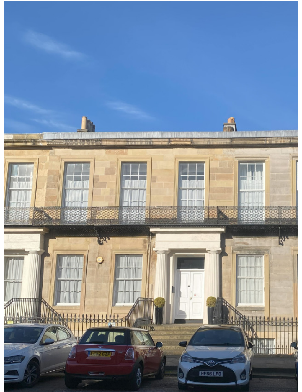
20 Windsor Street – Entrance Columns Painted
