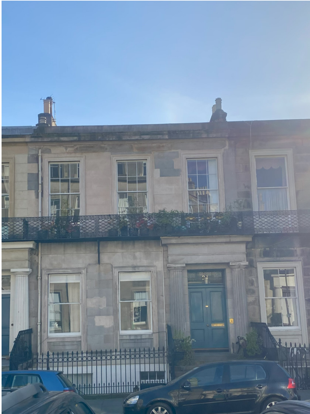
23 Windsor Street – Basement Wall Painted
