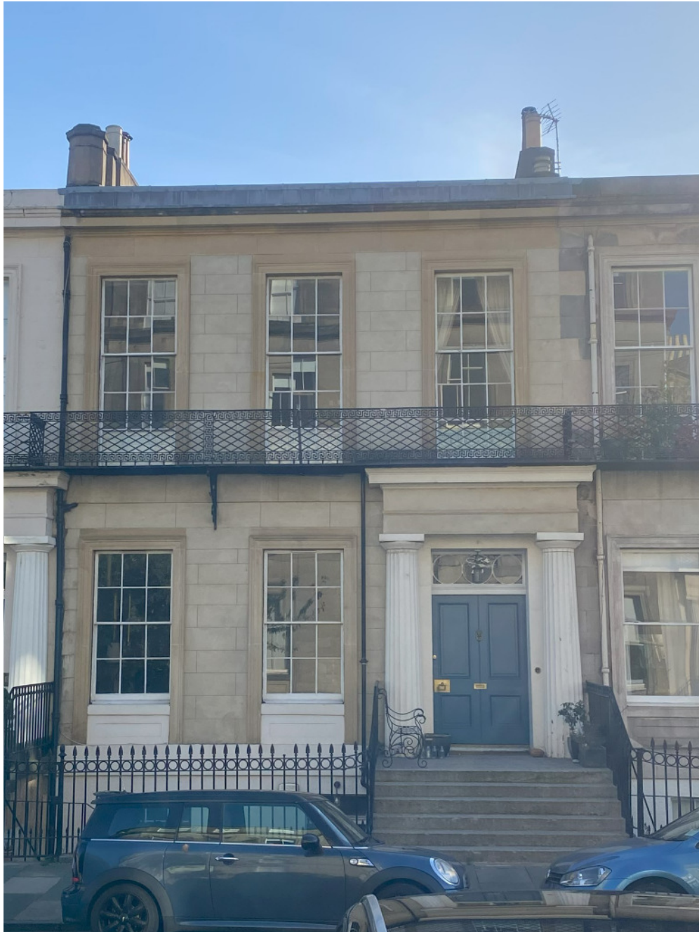
25 Windsor Street – Basement Wall, Entrance Columns Painted
