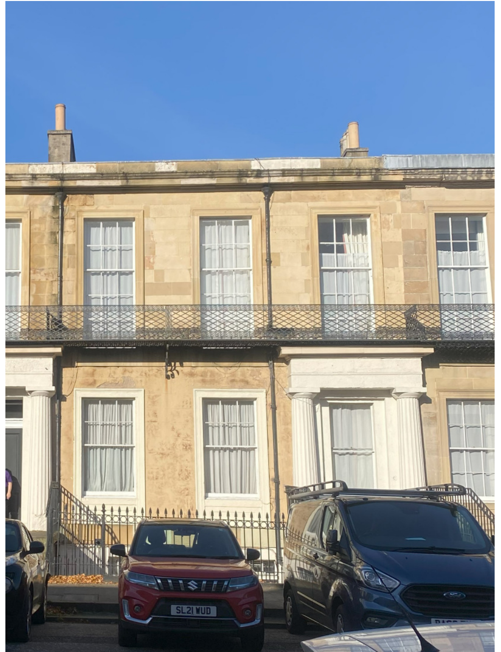
18 Windsor Street – Basement Wall, Entrance Columns & Window Reveals Painted
