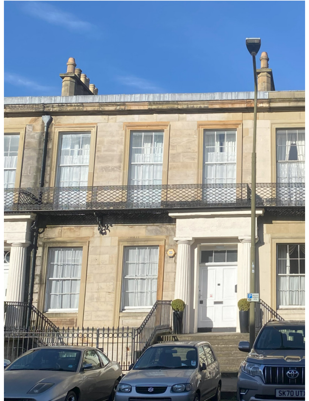
24 Windsor Street – Entrance Columns Painted
