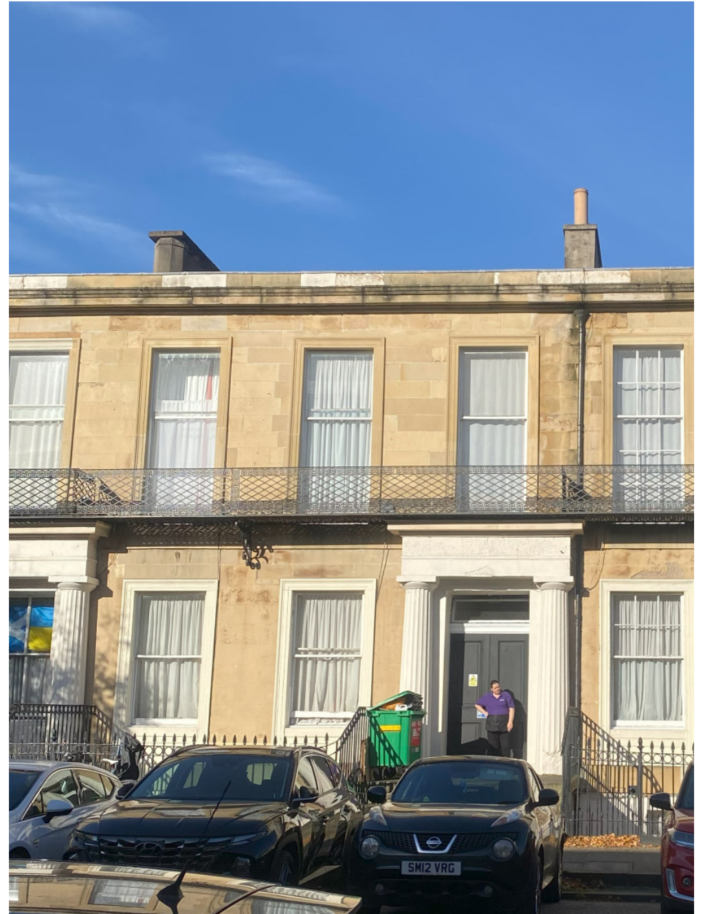
16 Windsor Street – Basement Wall, Entrance Columns & Window Reveals Painted
