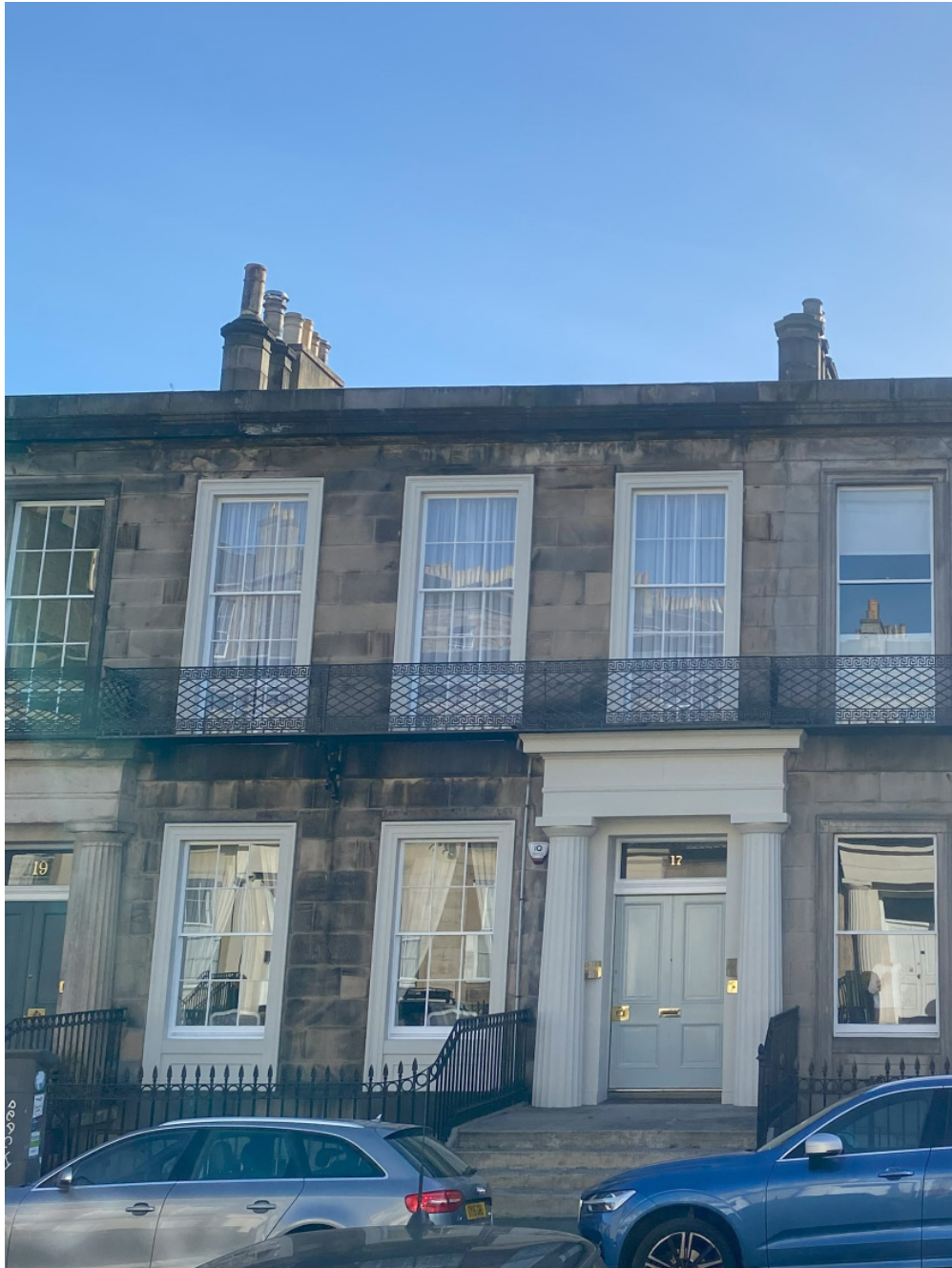
17 Windsor Street – Entrance Columns & Window Reveals Painted
