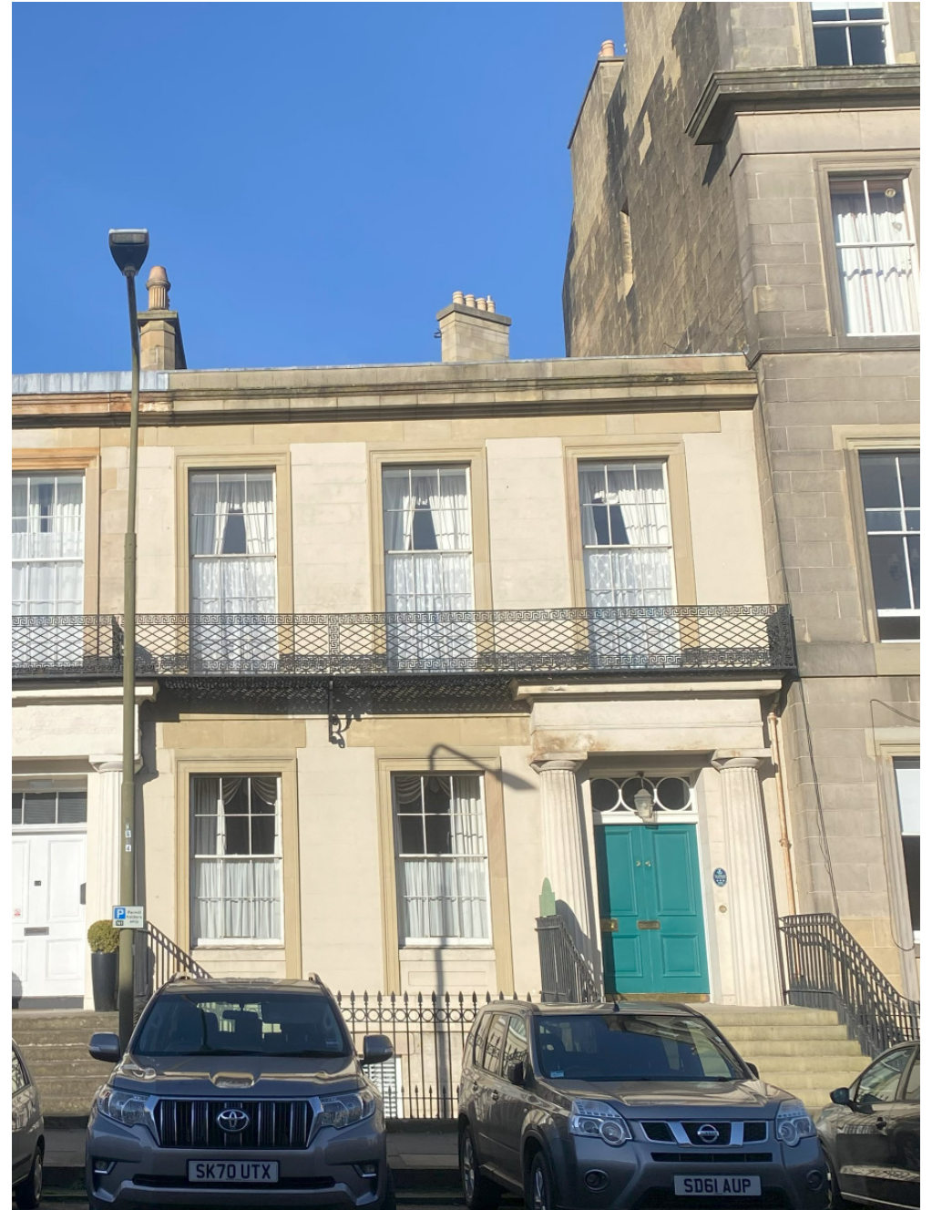
26 Windsor Street – Upper Elevation & Columns Painted
