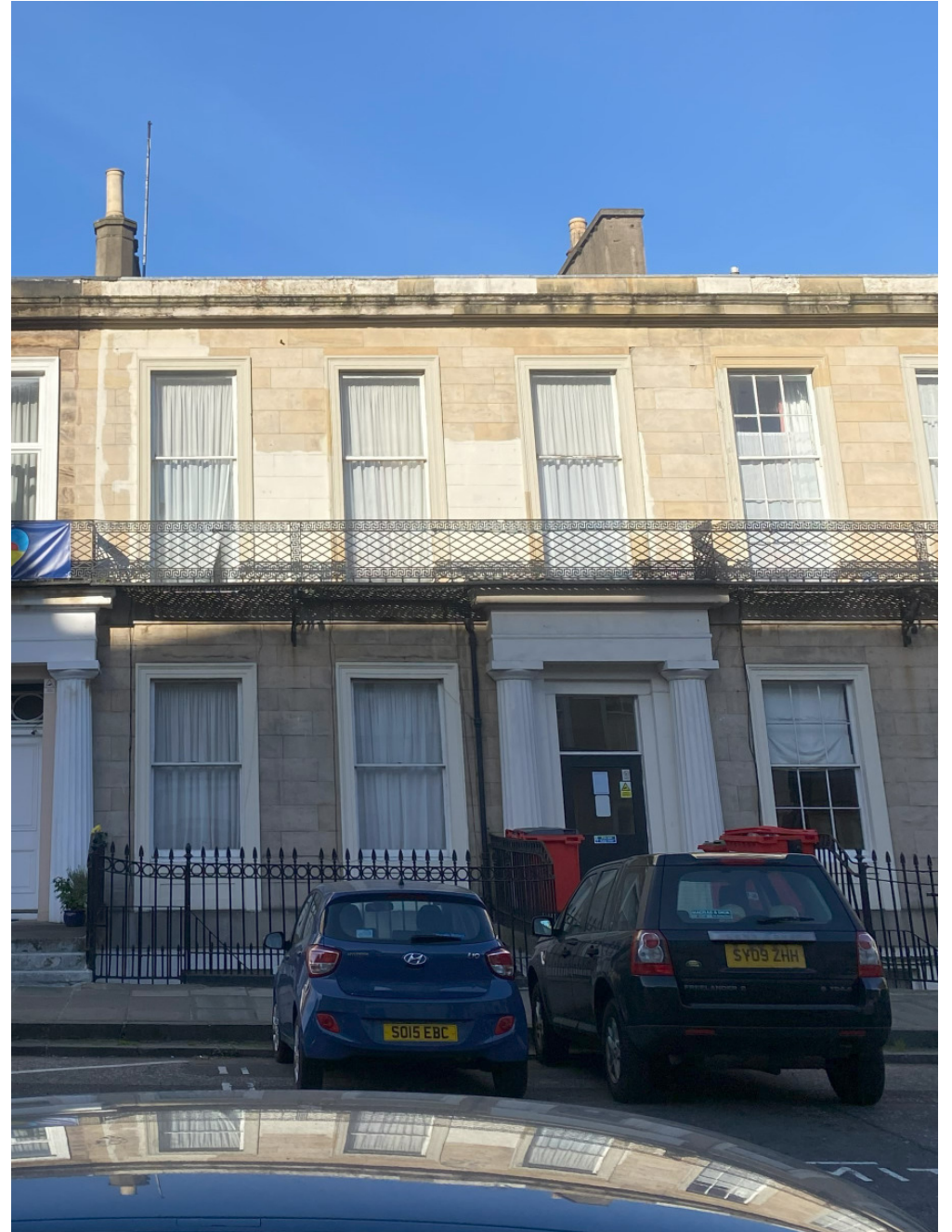
10 Windsor Street – Basement Wall, Entrance Columns & Window Reveals Painted
