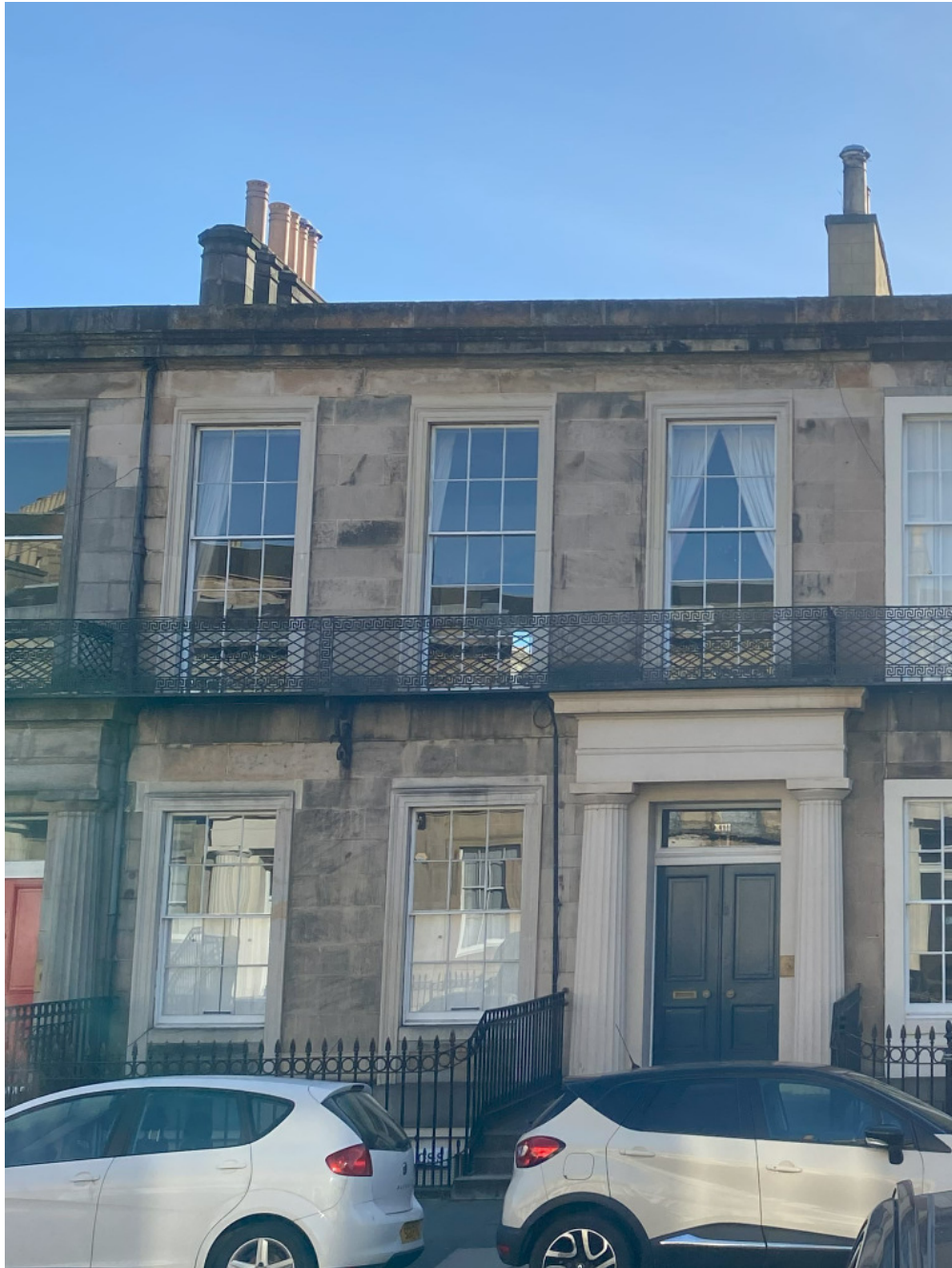
13 Windsor Street – Basement Wall, Entrance Columns & Window Reveals Painted
