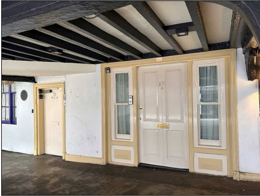
12a / 12 b Bridge Street Row The residential entrance to two apartments
