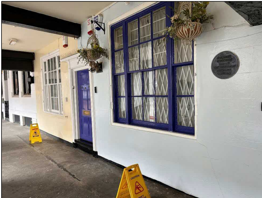
14/14a Bridge Street Row Ditto.
