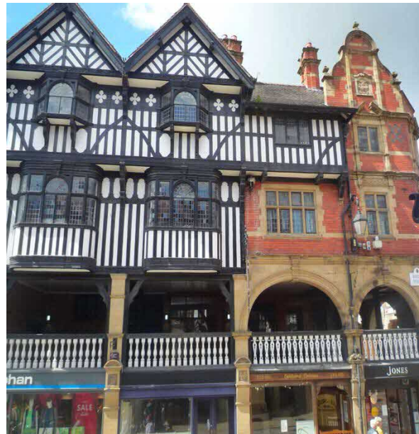
Fig 3. Bridge Street West, adjacent to the Cross, built by Lockwood in 1892.
