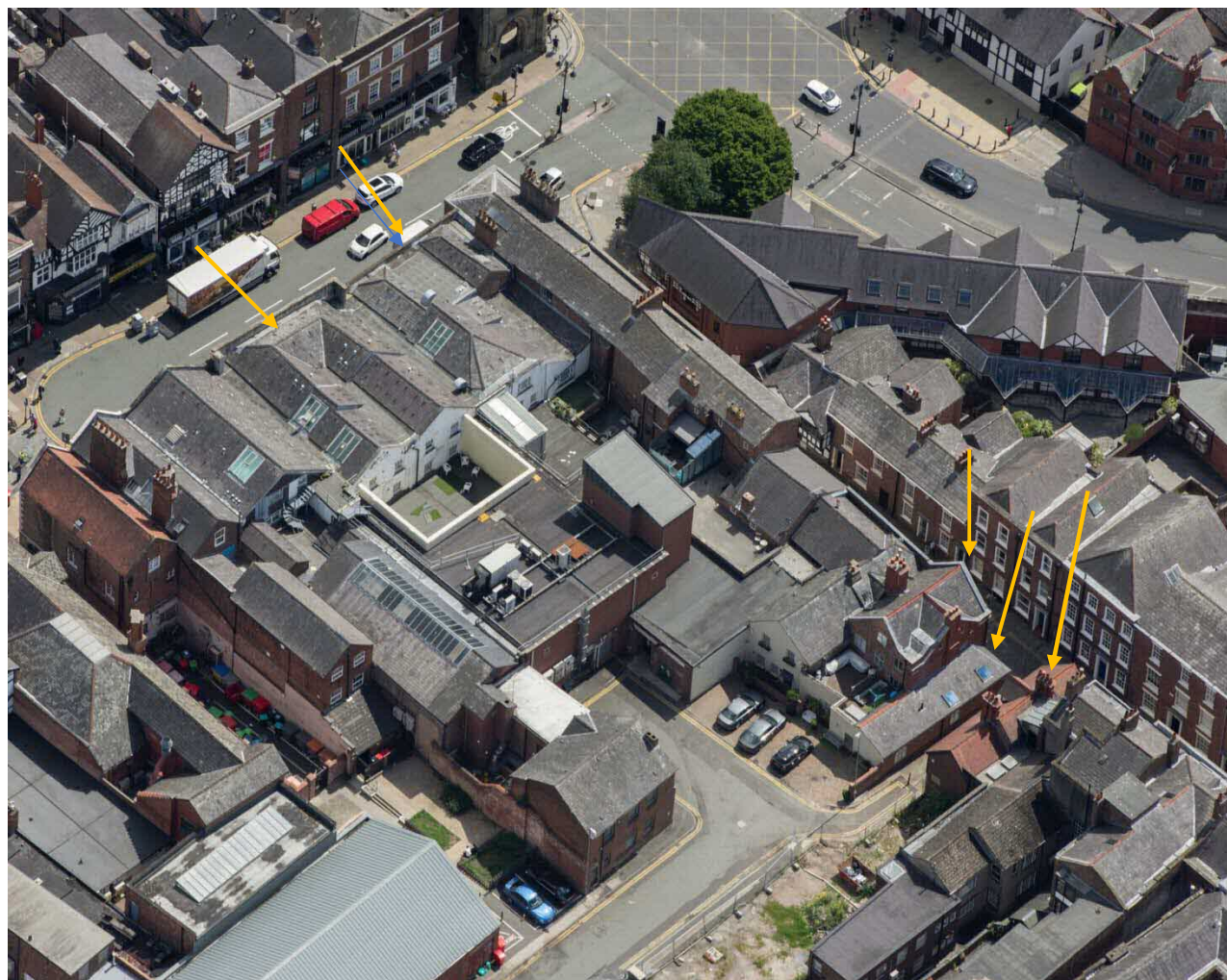
Fig 21. Aerial photo of White Friars and the rear of Bridge Street. Note roof terraces in the vicinity arrowed in yellow. All of these are listed buildings.
