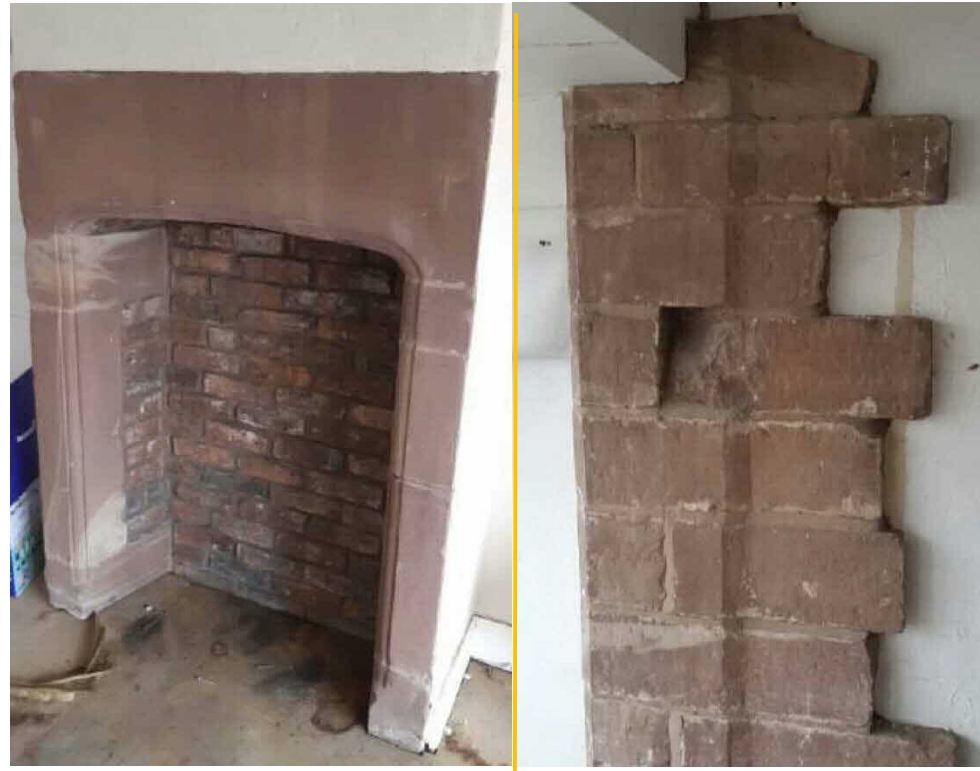
Fig 7. Left: The 17 th century sandstone fireplace on the Row plus two level; Right The 17 th century sandstone piers to north and south walls with lamb's tongue stops.
