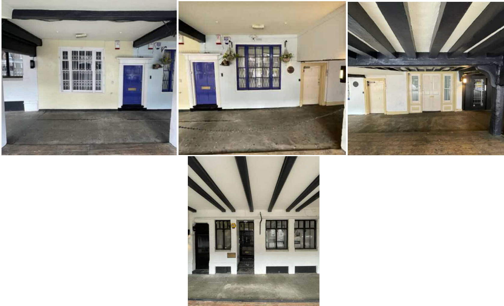
Fig 18. Domestic frontages on Bridge Street West
