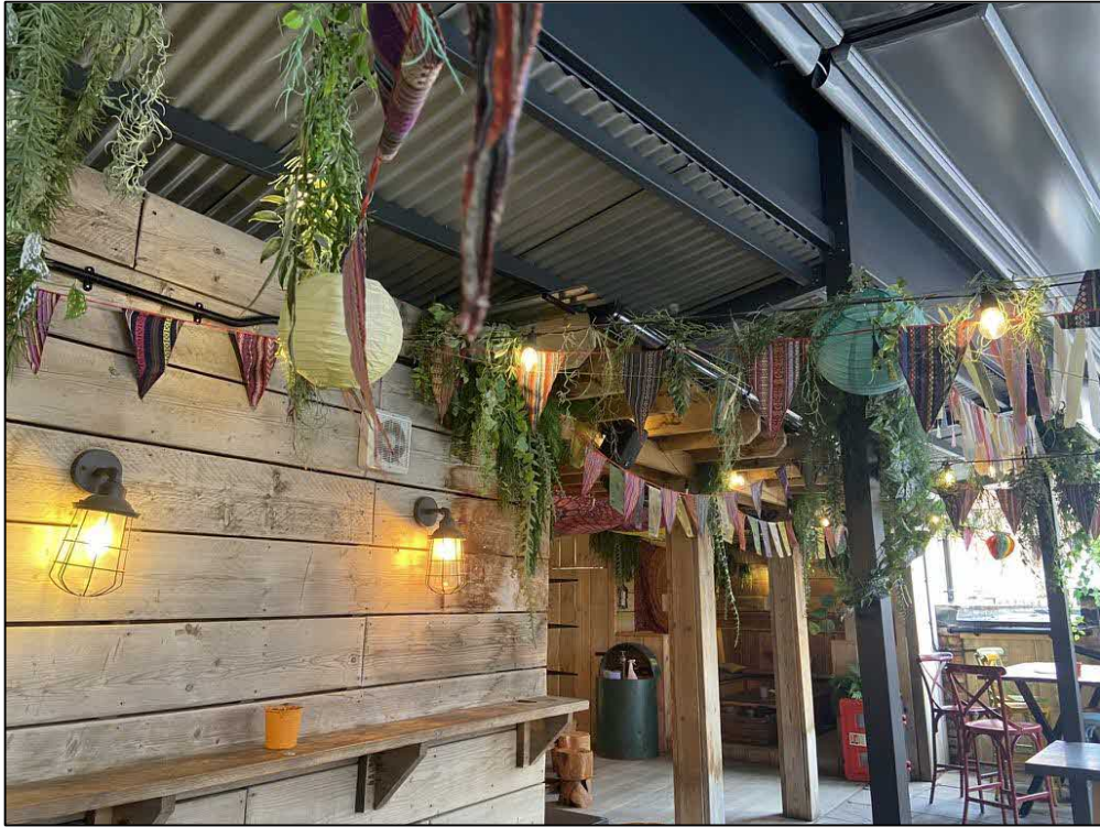
Fig 10: Another section that is to be removed (Building labelled C). The building is a timber construction with a corrugated tin roof. Again, erected not long ago to support the adjacent active bar, this building is utilised as an outdoor terrace shelter.
