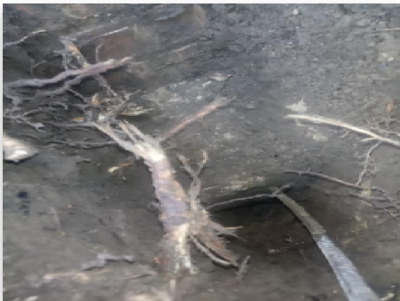
Fig 1.3: Trial Hole 1 Footing
