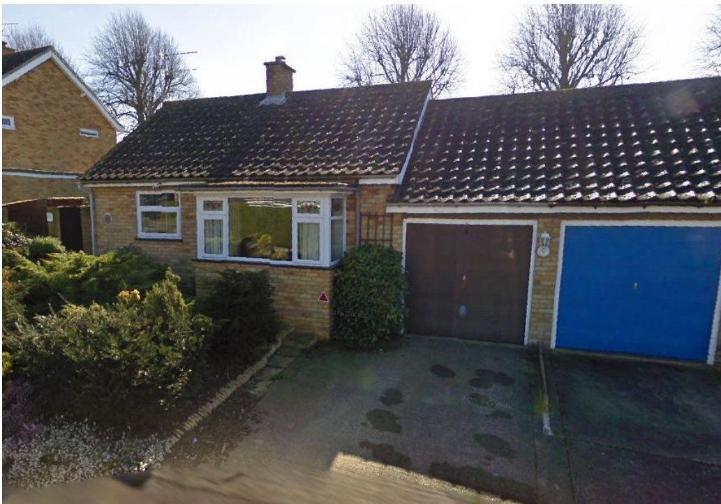
Front elevation of the property and garage, with the trees shown to the rear.
