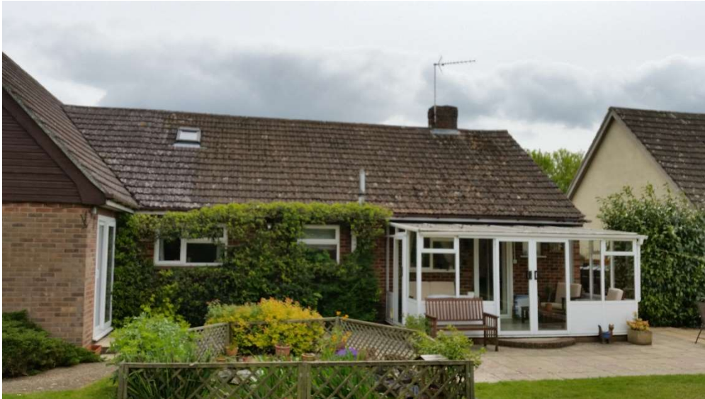
View of the rear elevation and conservatory from the north east
