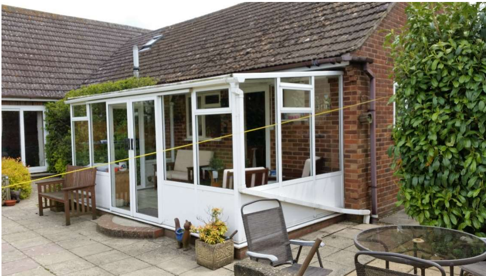
View of the rear elevation and conservatory from the south west
