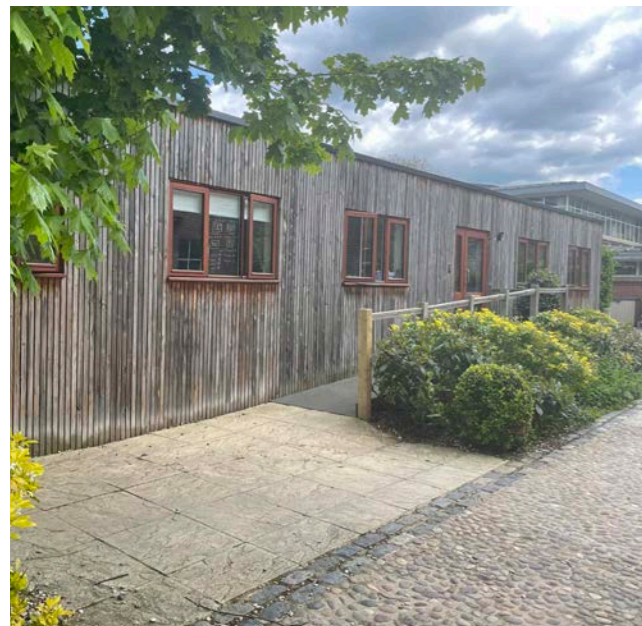
- Photograph of West Elevation
