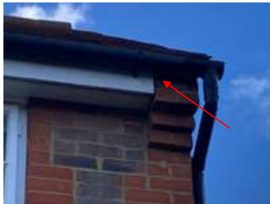
Photograph 6: Gap between soffit and brick
