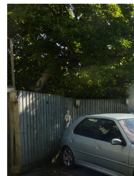
Mounted light fittings on existing close board fence
