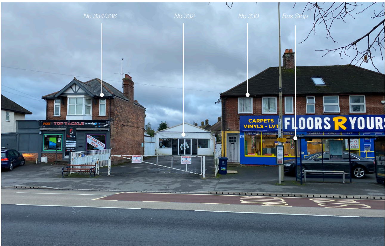
Existing Abingdon Road street frontage
