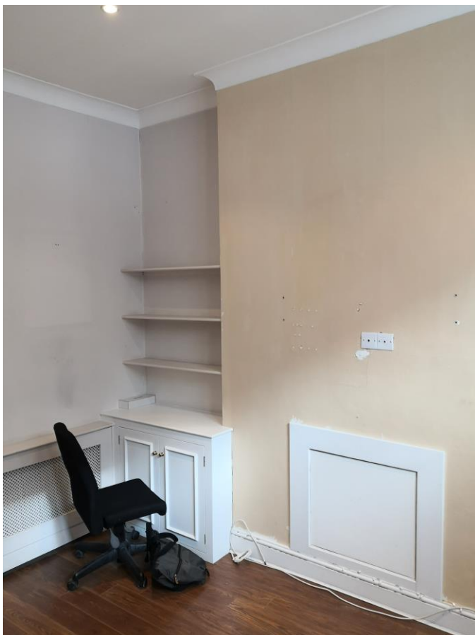
Ground floor front room, showing absence of original ornamentation
