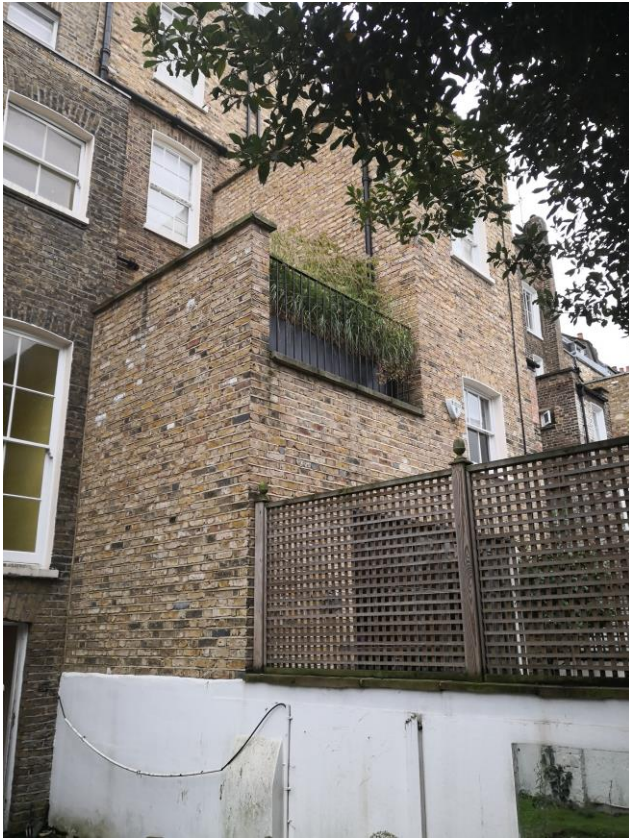
Rear extension to 100 Ebury Street adjoining
