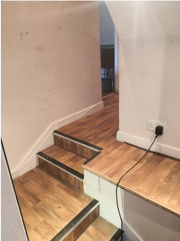
New staircase to lower ground floor
