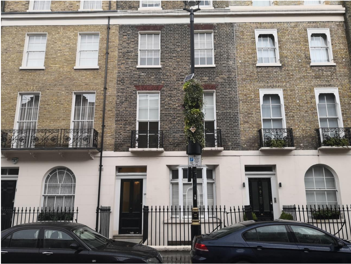
Front elevation of property, showing modern bay window
