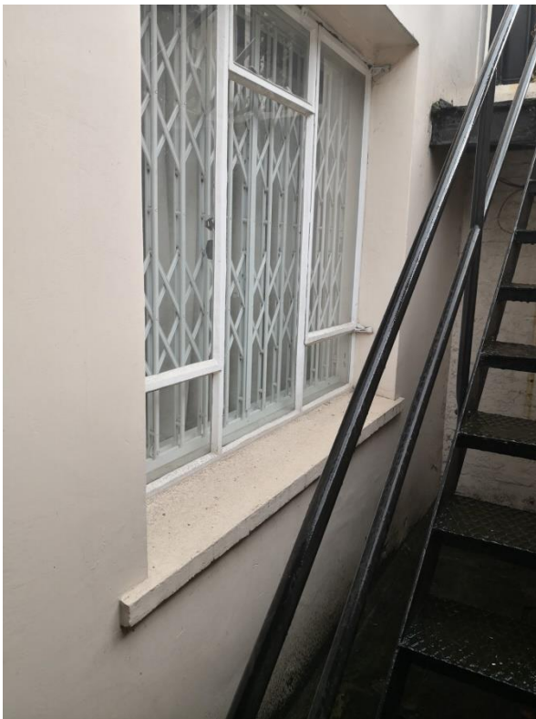
Modern window to lower ground floor front elevation
