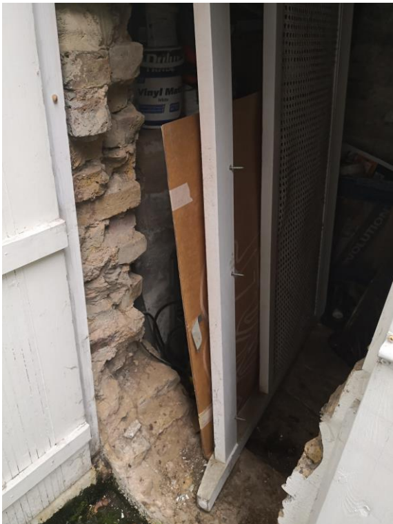
Blocking of vault to rear of property (top) and new opening to vault (bottom)
