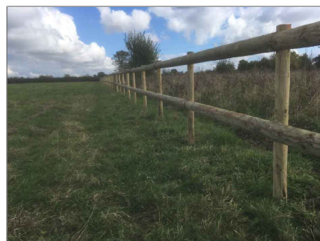
2 RAIL, HALF ROUND, POST AND RAIL FENCING
