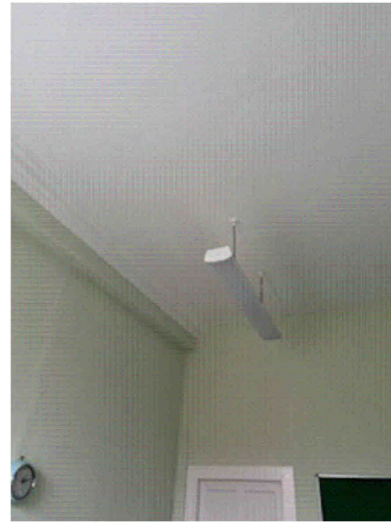
Room 211 South west corner ceiling bulkhead/ cornice all retained
