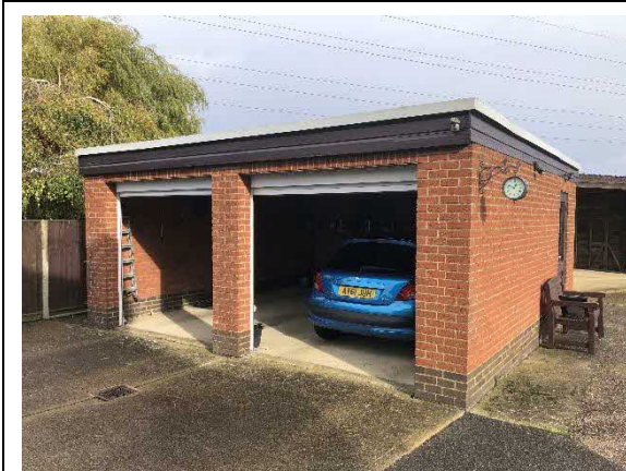
Garage building to be demolished.
