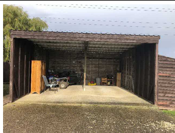
Storage building to be demolished.
