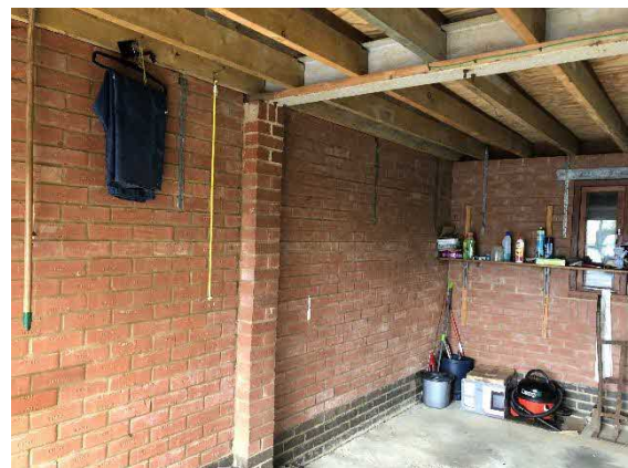
Interior of the main garage building.
