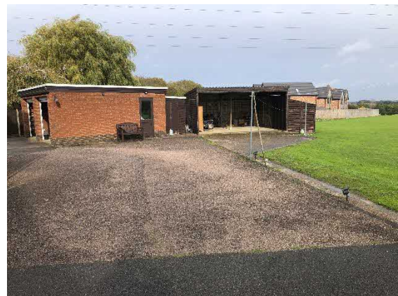
Photo of entire works area.
