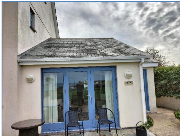
The building viewed from the western aspect.
