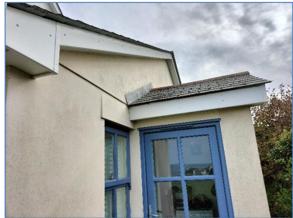
The small porch extension.
