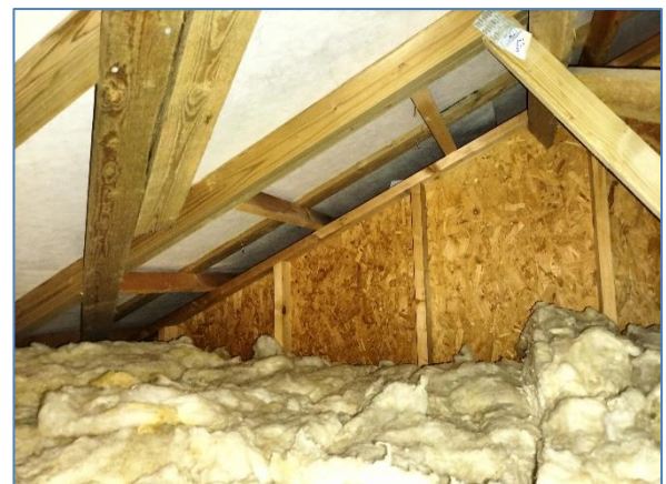
The roof void
