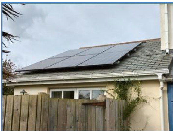
The eastern aspect of the roof
