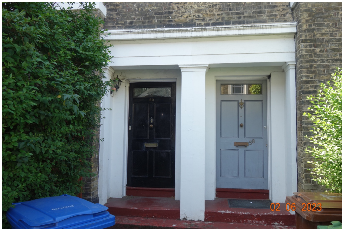
Image 5 Porches to 58 and 60 showing clearly the Greek character of capitals and cornice.
