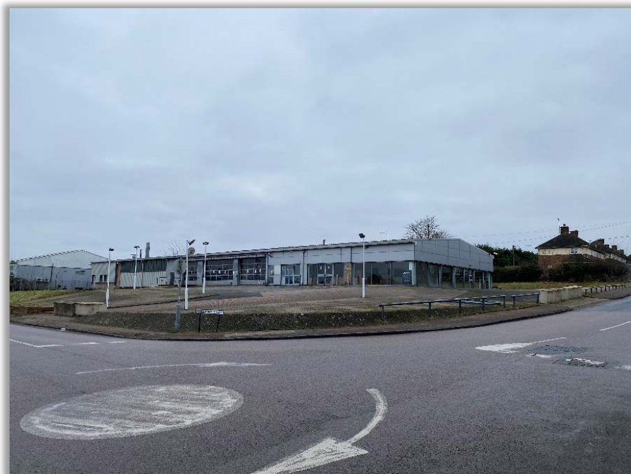
Figure 4 – View towards the site from junction of Duddery Hill and Hollands Road
