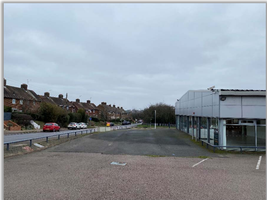
Figure 10 - View of front of site looking north-east
