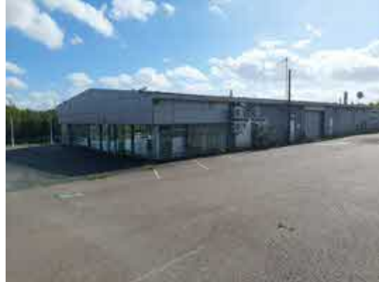
Photograph 2: Western elevation of building B1.
