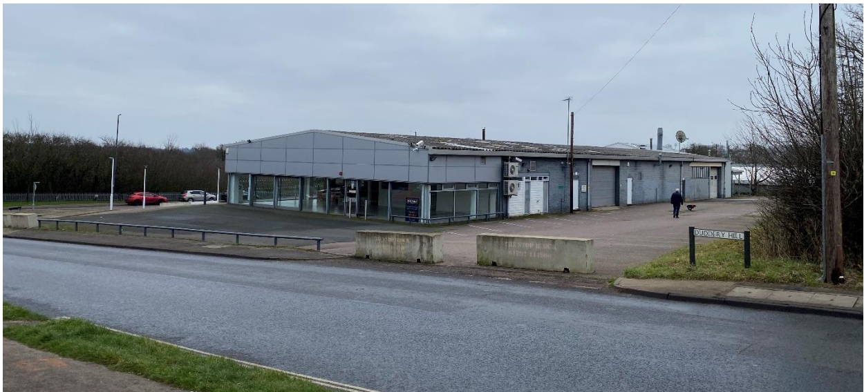
View from Mill Hill. (Photograph prior to demolition, for reference).
