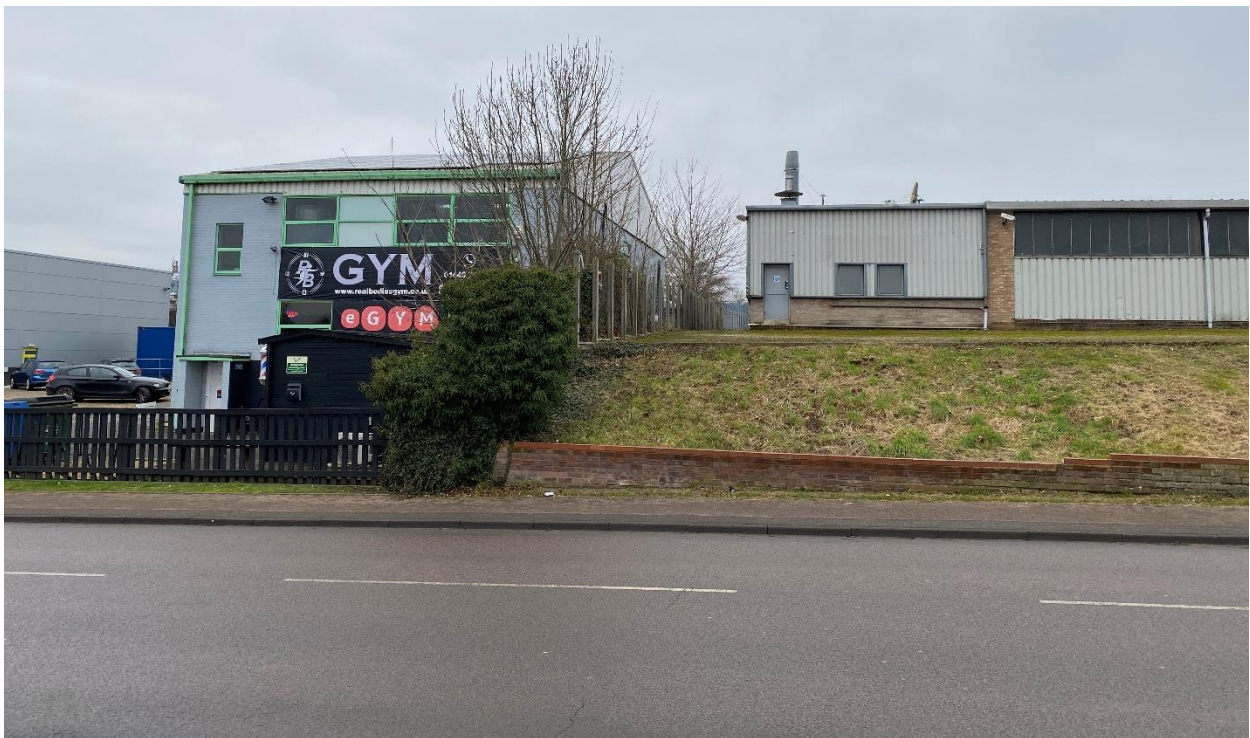
South end of the site on Hollands Road with neighbouring Gym some 4m lower than the application site, and showing the brick wall and steep grass bank. (Photograph prior to demolition, for reference).
