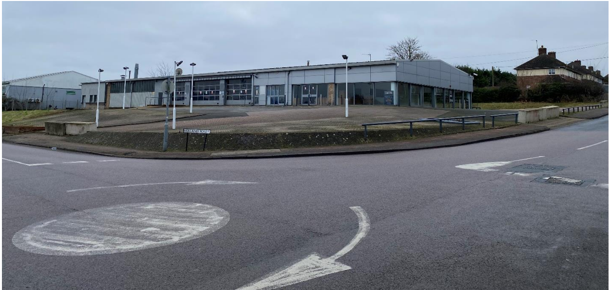
West side from Doddery Hill at junction with Hollands Road. (Photograph prior to demolition, for reference).
