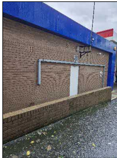
Building TN3 (West elevation)
