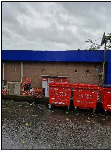
Building TN3 (North elevation)
