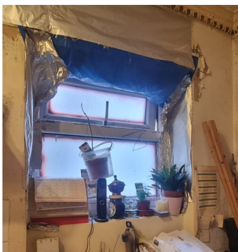
Interior View of the Existing uPVC Window
