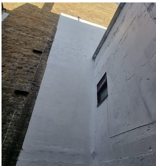
External View of the Existing uPVC Window
