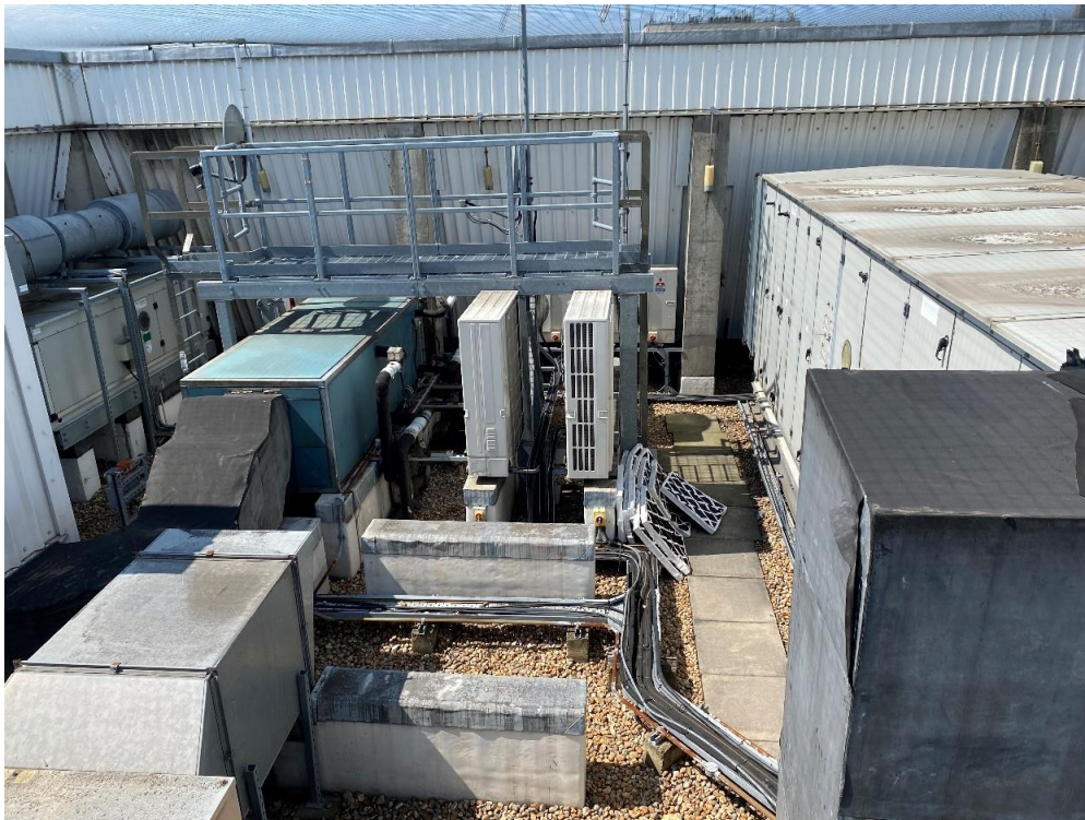
PHOTOGRAPH 4: Roof level plant area.
