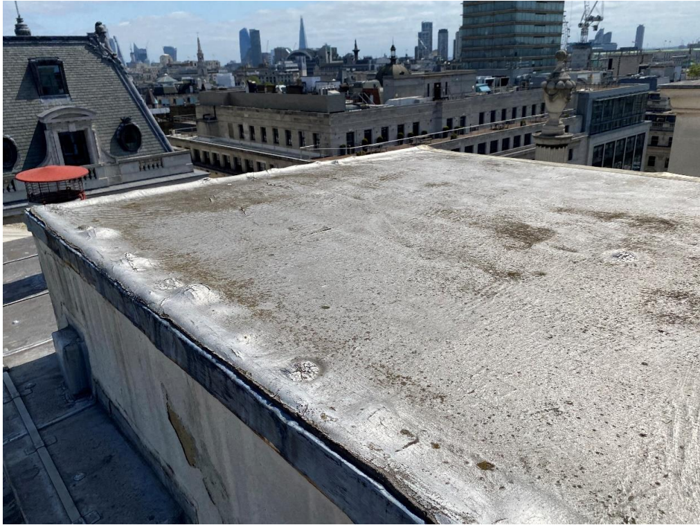
PHOTOGRAPH 7: Asphalt covering to flat roof area.
