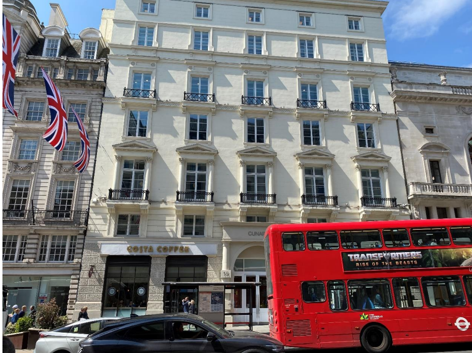
PHOTOGRAPH 1: General View front elevation.
