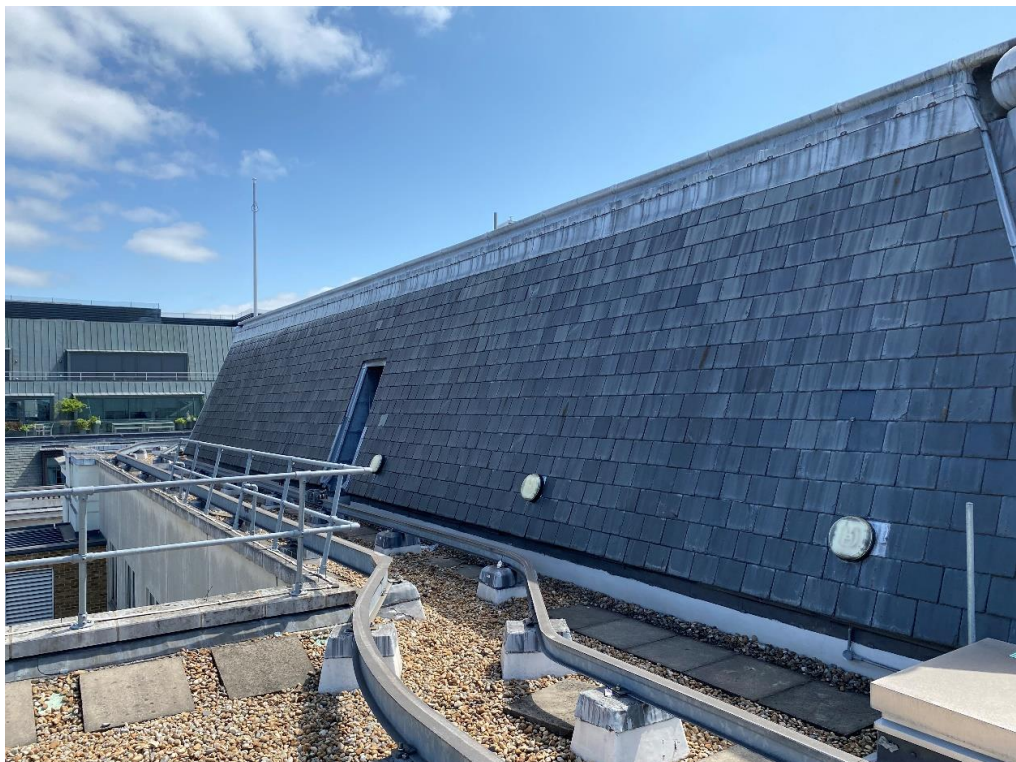
PHOTOGRAPH 6: General roof area.
