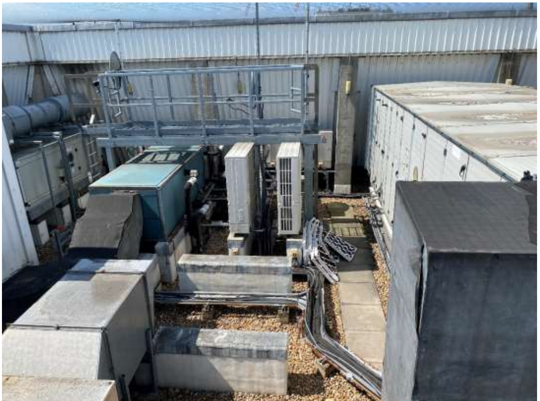
Photo 4: Roof level plant area.
