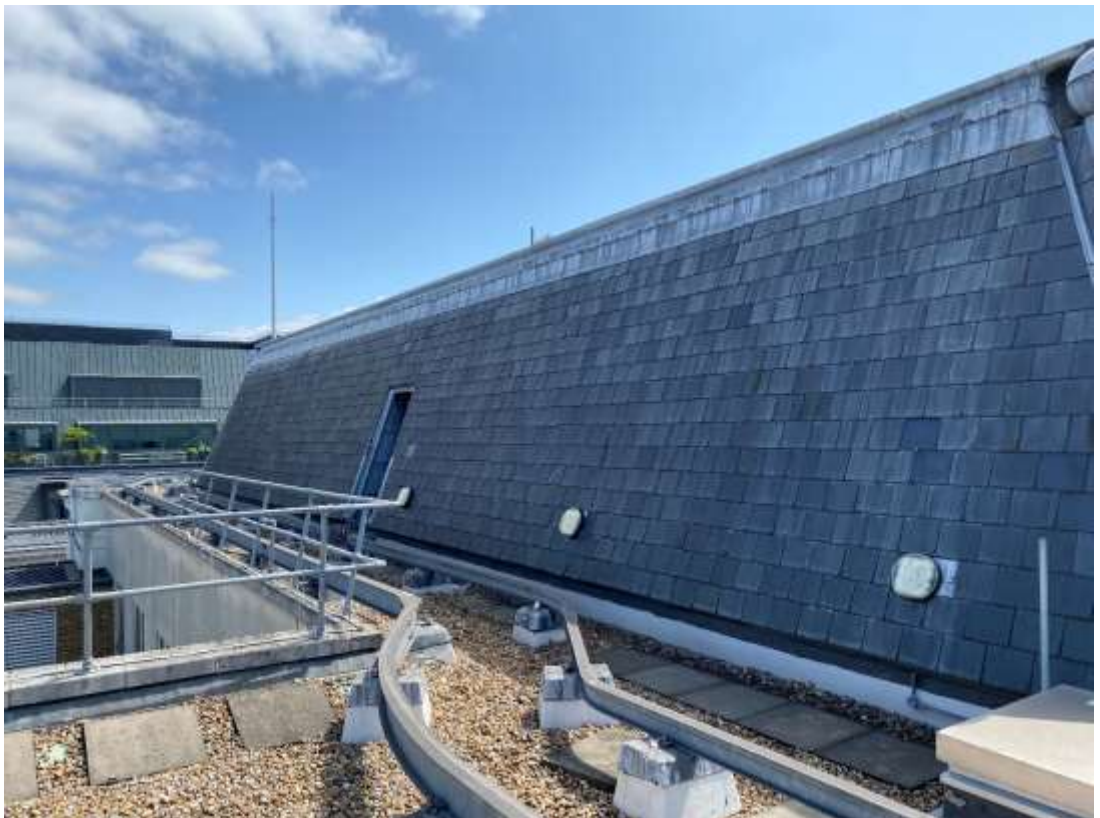
Photo 6: General roof area.
