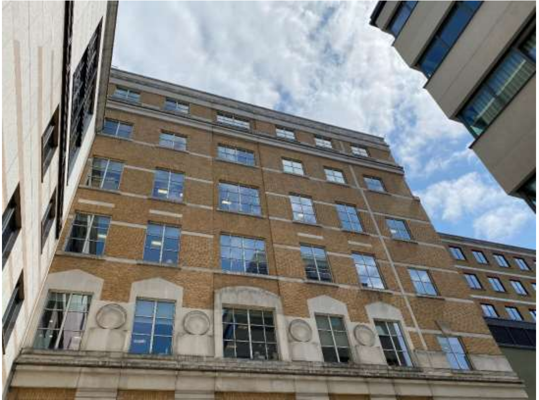
Photo 3: Rear elevation high level.
