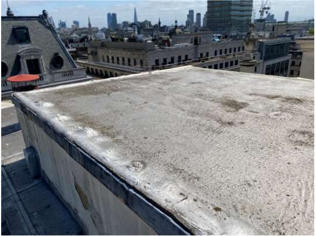
Photo 7: Asphalt covering to flat roof area.
