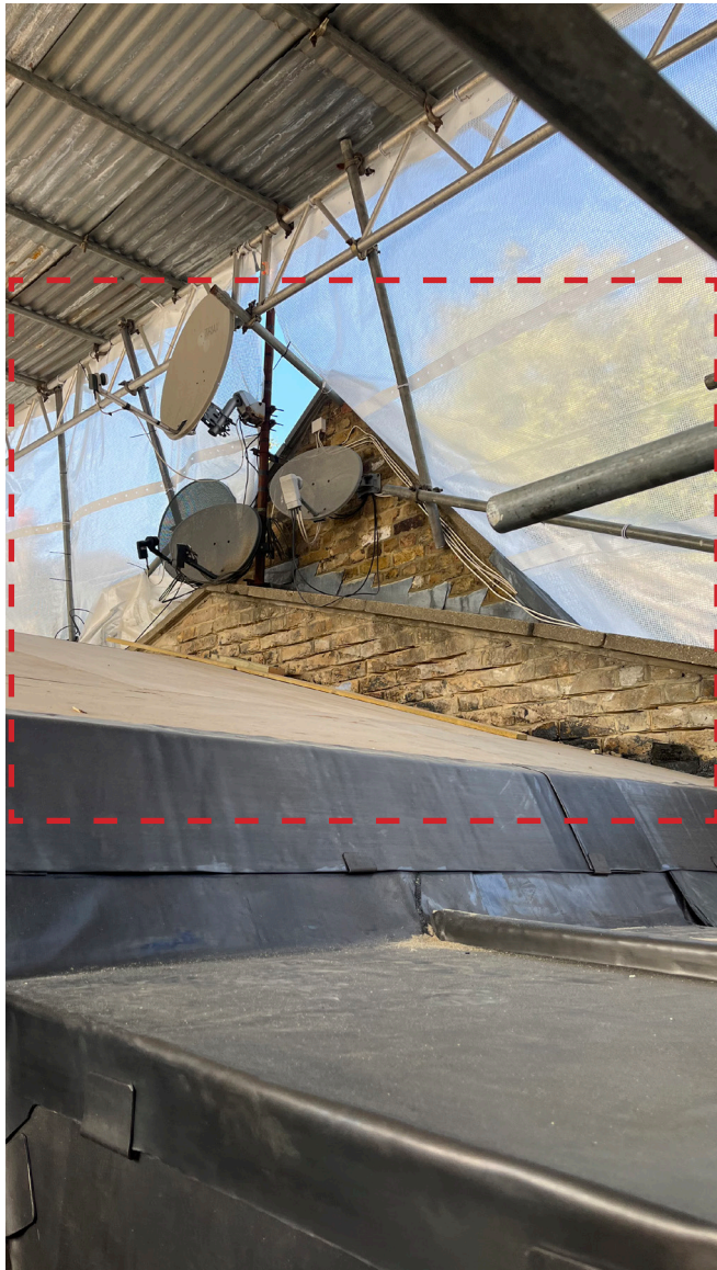
Existing roof & neighbours wall
